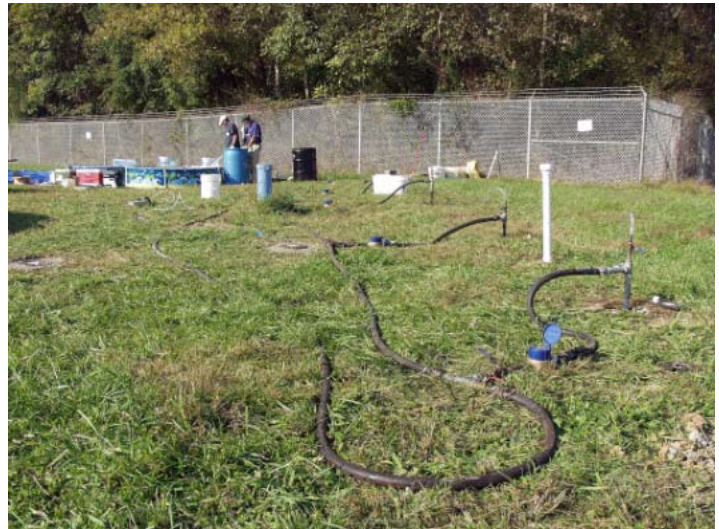
PHOTOGRAPH 2 Injecting EOS ® at the Maryland site.
