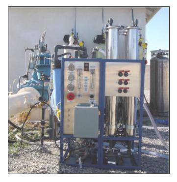
Photograph 2: Watts Premier M-15,000 RO Treatment System at CVWD Well 7802
