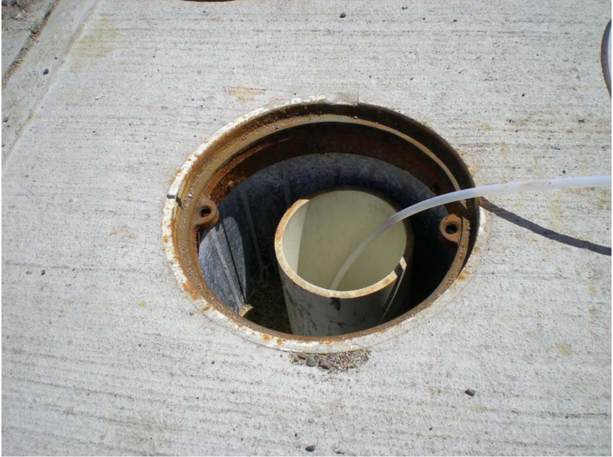
Picture 8. Normal monitoring well completion.
