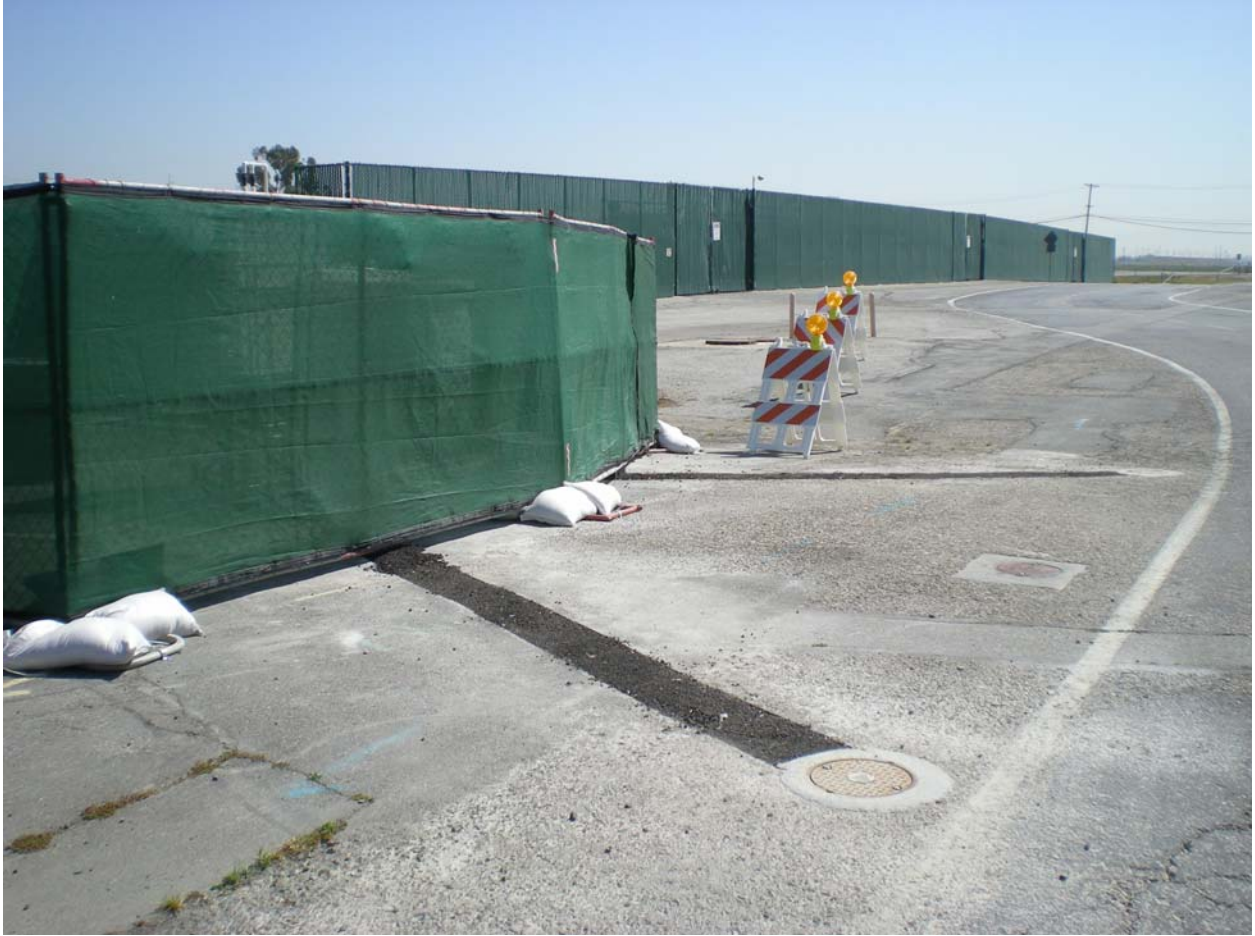
Picture 7. Extraction well trench.
