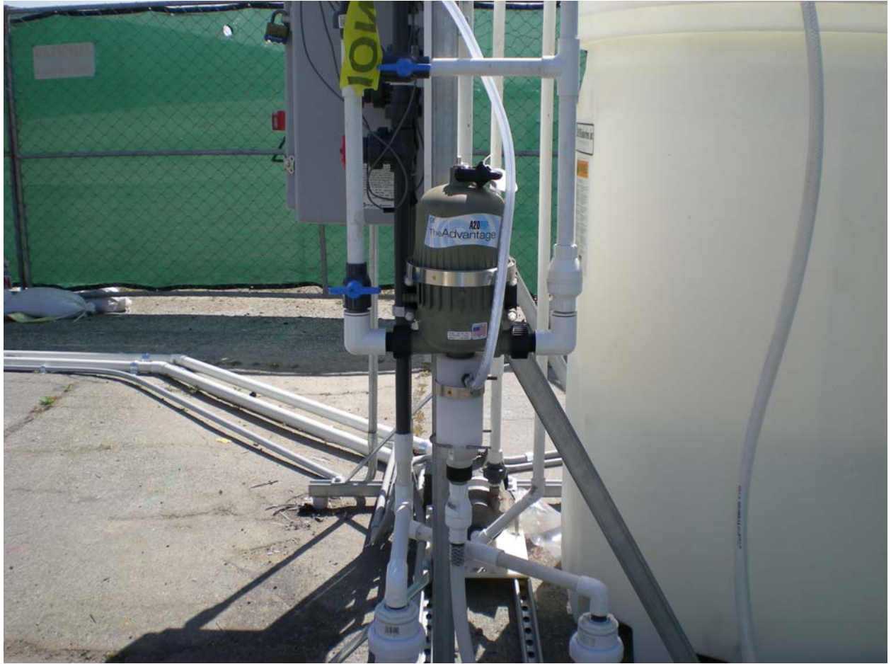
Picture 4. Dosatron setup.
