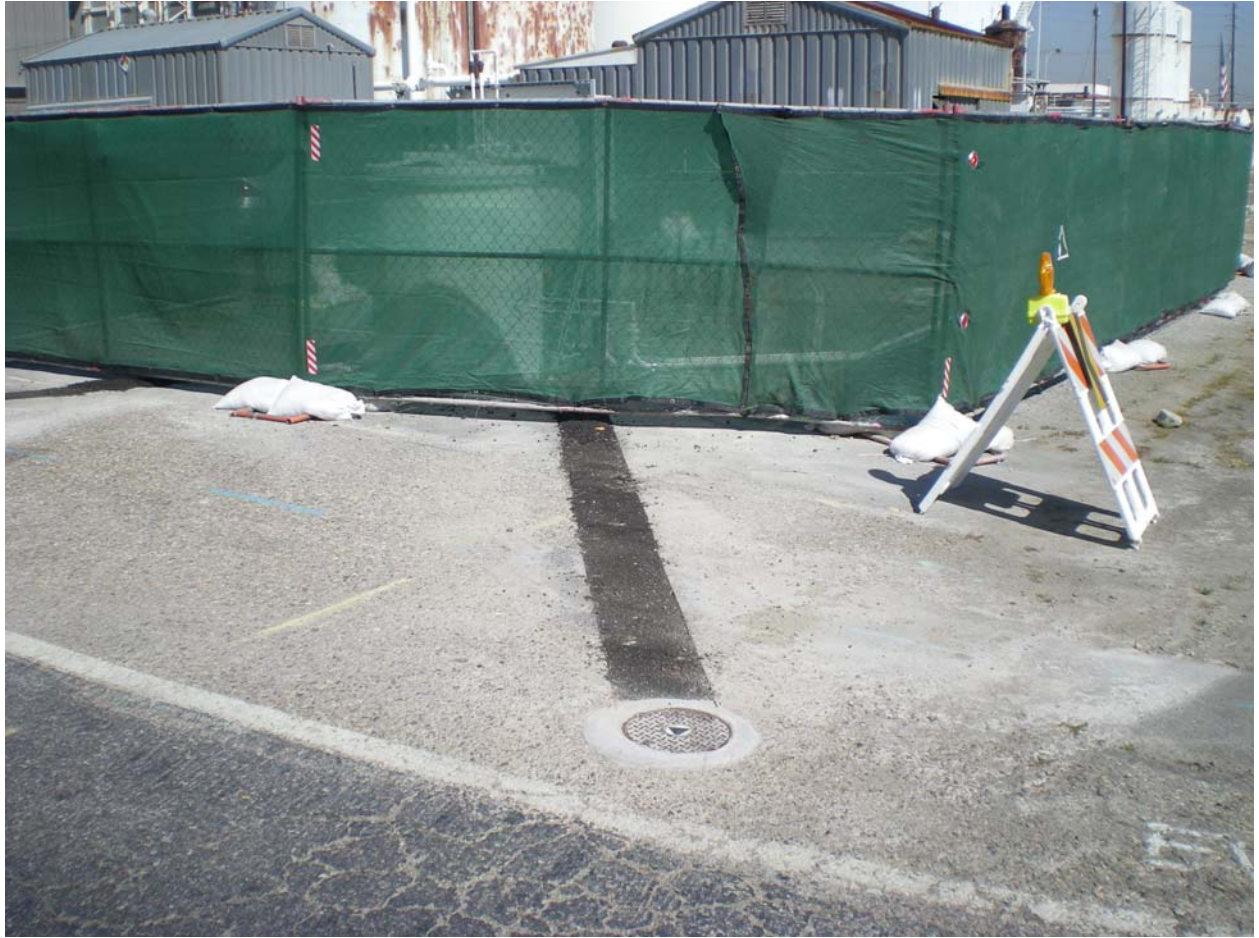
Picture 22. Treatment compound area.
