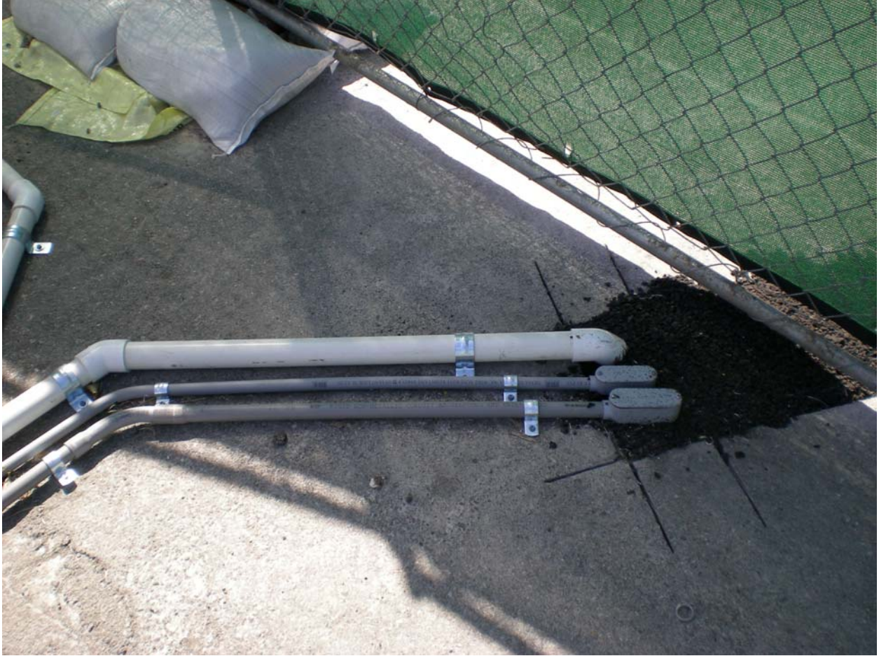
Picture 6. Extraction piping daylighting.
