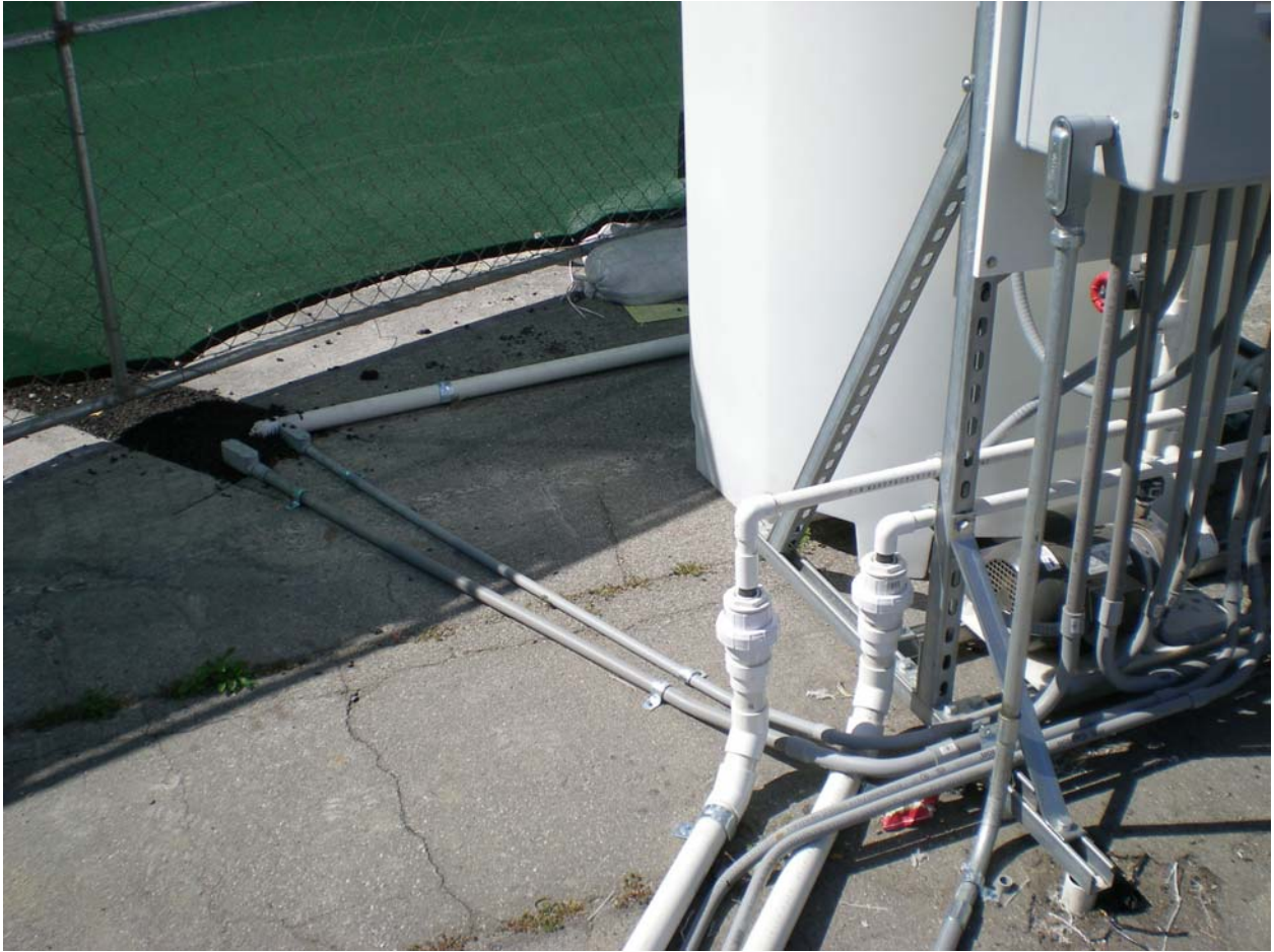
Picture 5. Extraction piping daylighting.
