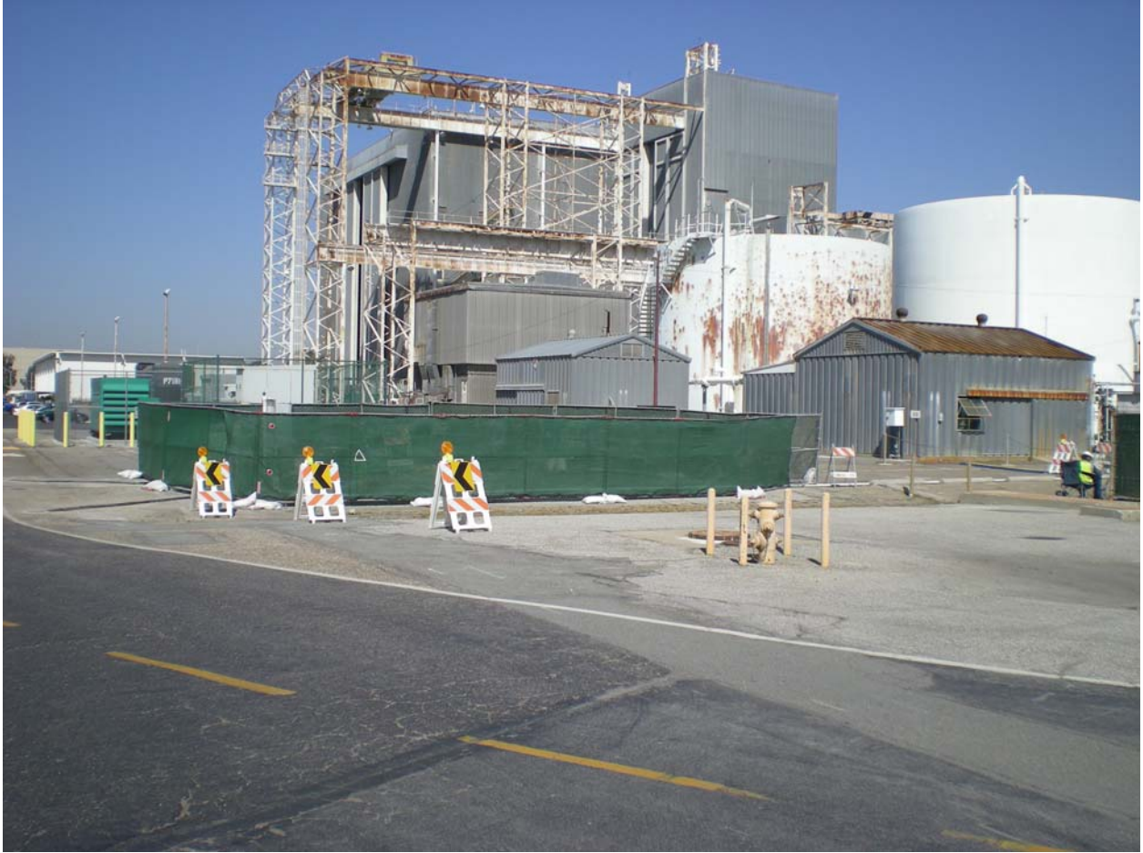
Picture 21. Treatment compound area.
