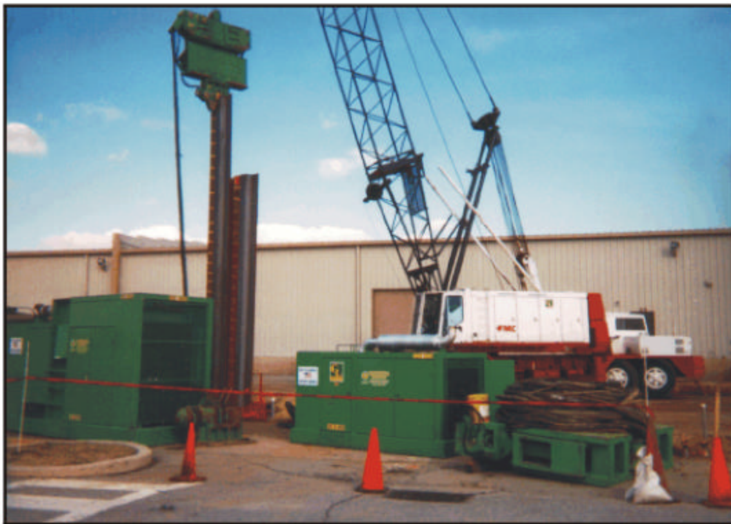
Figure 7-9. Sheet Piles Installed Using a Vibrating Hammer
