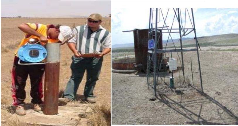
Manual/Automatic Groundwater Monitoring
