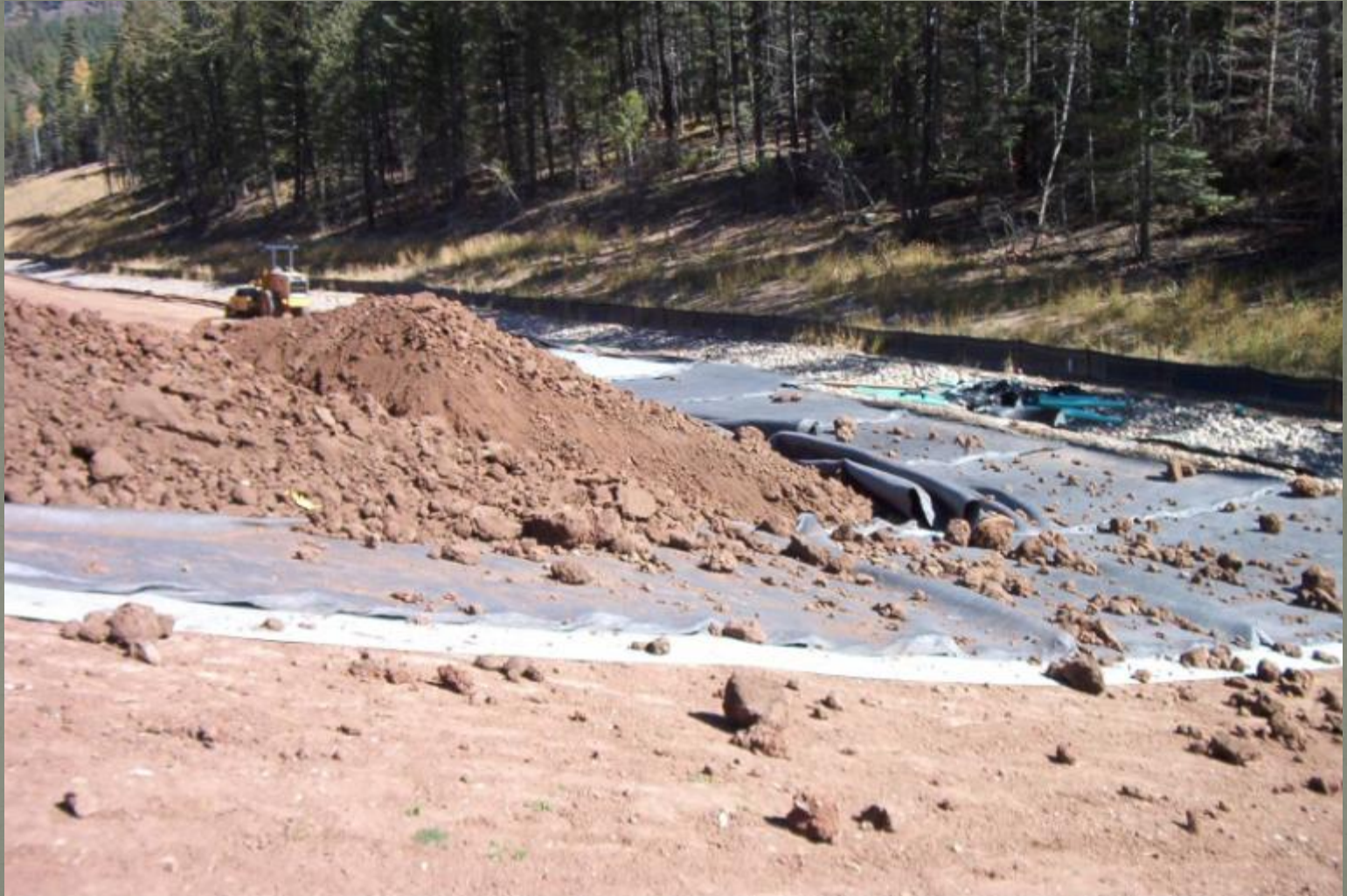
Slope Instability with GCL (Interface Friction)
