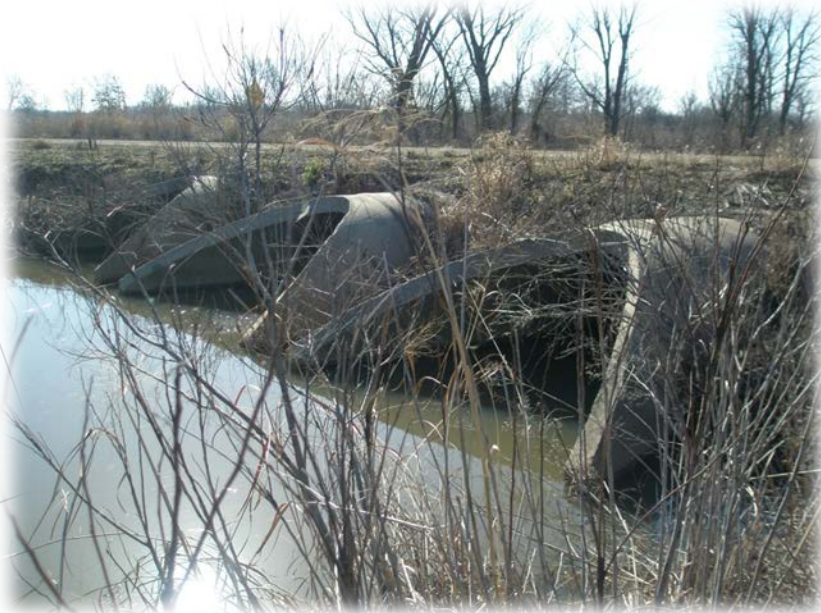
Tar Creek - SW Star Road Culverts Southwest of Muncie Pit
