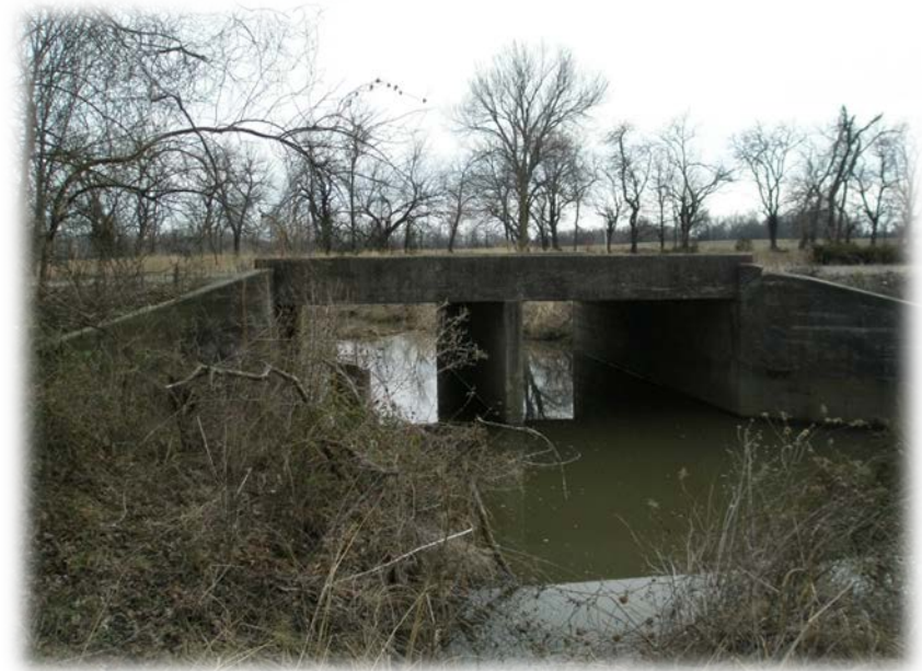
Northwest Tributary - SW Star Road Culvert Southeast of TC-2
