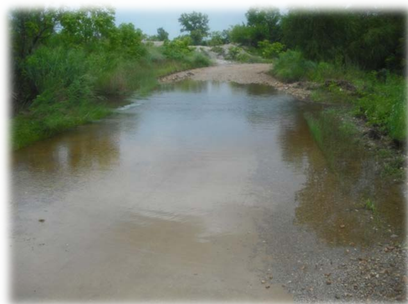
State Line Road Low-Water Crossing
