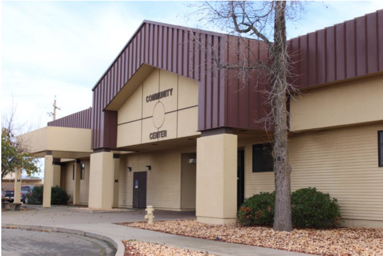
Figure 3. Beale AFB Community Activity Center (CAC), Building 2425. (Picture from the Beale Force Support Squadron website at http://www.bealefss.com/community-center/ ).
