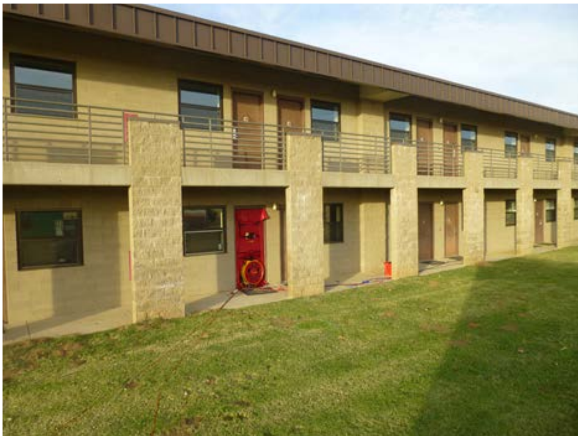
Figure 3. Beale Air Force Base Building 24176 (Dormitory Building B).
