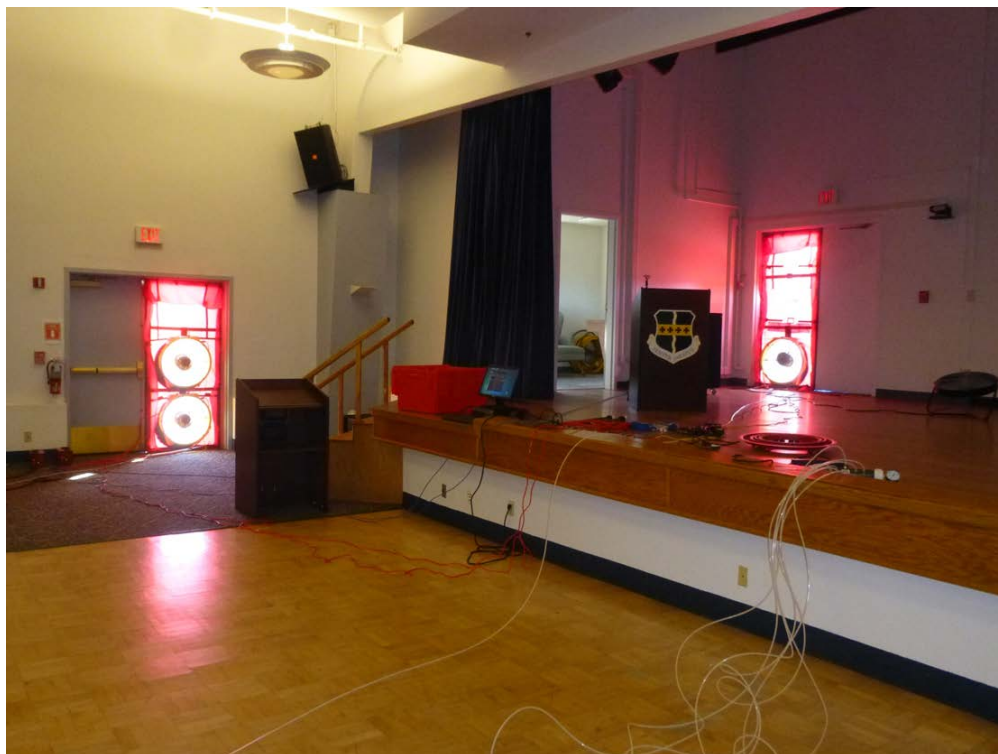
Figure 8. Blower door installation and the use of floor fans to facilitate air mixing near the blower intake sampling area.
