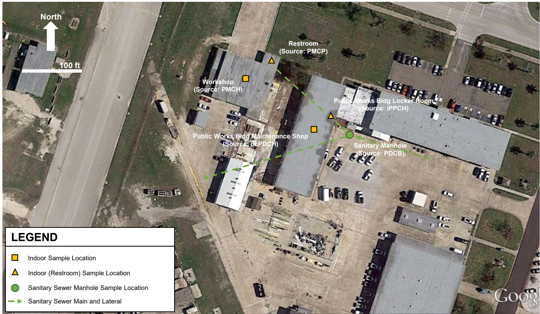
FIGURE C.9 TASK 2 TRACER TEST: OFFICE AND SHOP BUILDINGS NASCC Area 3, Corpus Christi, TX October 2017
