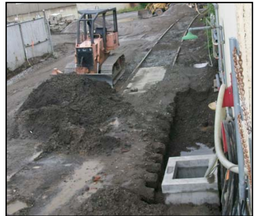
Figure 3. Electrode placement below railroad spur and building.
