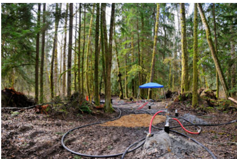
Figure 3. Electron donor injection to multiple wells within a row.
