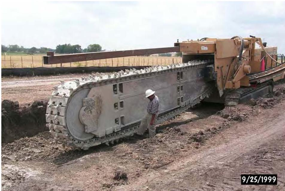
**Figure 2.2 Rock Trencher Employed at NWIRP McGregor, Texas**
