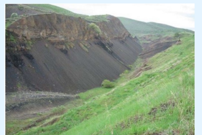
An ET cover was constructed on more than 500 acres where mining-related waste rock remains in place at the Ballard Mine Superfund site near Soda Springs, Idaho. The cover system was designed to slow the flow of stormwater runoff and limit soil erosion. Its vegetation layer enables significant sequestration of atmospheric carbon.
