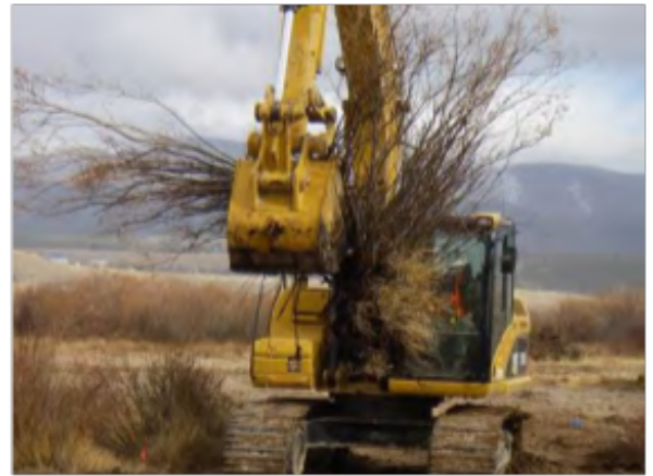
Healthy willows from distant parts of the floodplain were salvaged prior to full-scale application of soil amendments and transplanted along the river to help stabilize banks.
