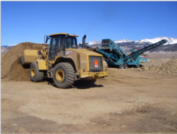
Rocks and soil were segregated for reuse in road construction and backfill.
