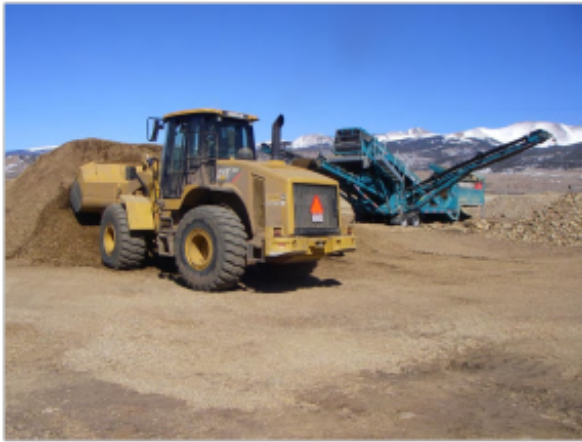
Rocks and soil were segregated for reuse in road construction and backfill.
