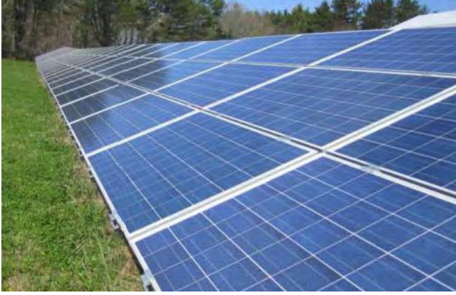
Solar Energy System: The onsite solar energy system consists of 644 PV panels configured in 46 groups operating in series and tied to the local utility grid. Capital costs for the PV system totaled approximately $772,000.
