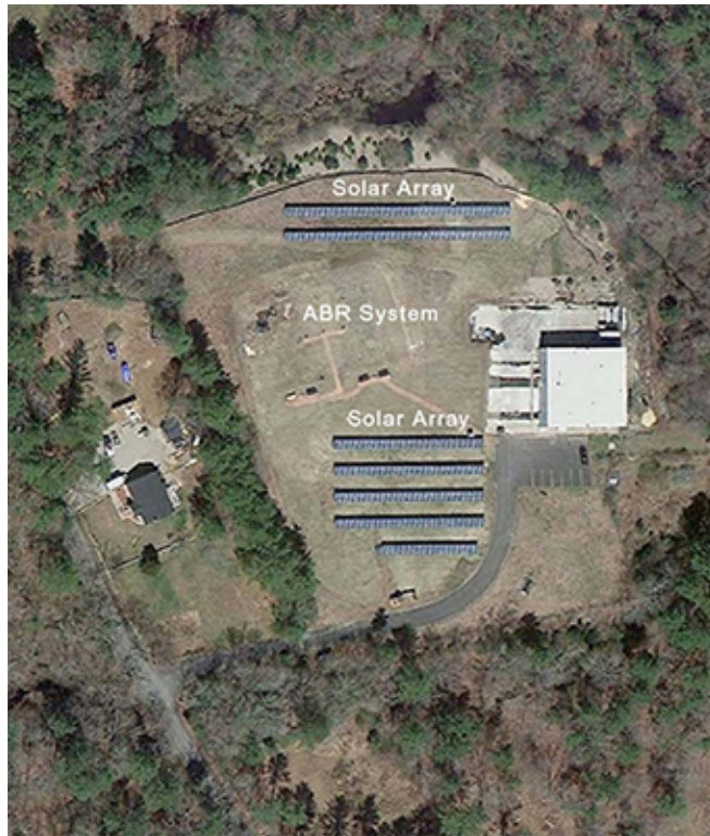
Aerial View: Proximity of the onsite bioreactor system, solar arrays and groundwater treatment building result in a relatively small surface footprint of cleanup activities.
