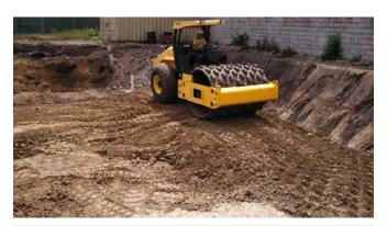
**Clay Barrier Installation:** Approximately 2,780 tons of clay, including 3 tons of bentonite, was compacted through use of a roller deployed in multiple rounds to achieve a 3-foot layer.
