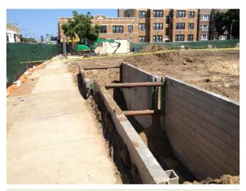
**ISCO** Reagent Mixing Trenches: The chemical oxidation reagents were mixed in three 16- by 16-foot trenches reinforced by steel. After mixing was complete, the steel was removed and reused onsite for purposes such as sidewalk shoring.
