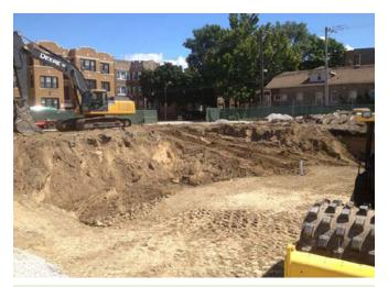
**Machinery Deployment:** Diesel fuel consumption and associated air emissions of machinery such as a 250-horsepower excavator and a 100-horsepower soil compacting roller were reduced through engine idle restrictions.
