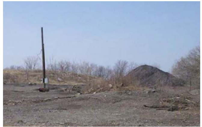
Soil Stockpiling: Soil excavated from the slag processing area was screened for lead content and segregated onsite in accordance with risk-based acceptable levels for industrial use. Slag waste with lead concentrations within the acceptable limits was stockpiled (as shown on right) for use as fill in onsite areas where land use is limited through institutional controls.
