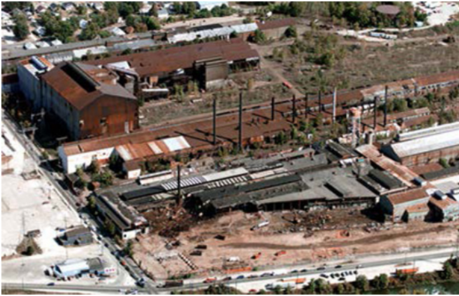
Prior to Demolition: From 1914 to 1986, the Continental Steel Corp. facility in Kokomo produced nails, wire and wire fence from scrap steel. Onsite manufacturing operations involved use, handling, storage and disposal of hazardous materials. The steel-making operations included material reheating, casting, rolling, drawing, pickling, galvanizing, tinning and tempering. The main plant area continues to be zoned for industrial use. (photo source: Kokomo Tribune)
