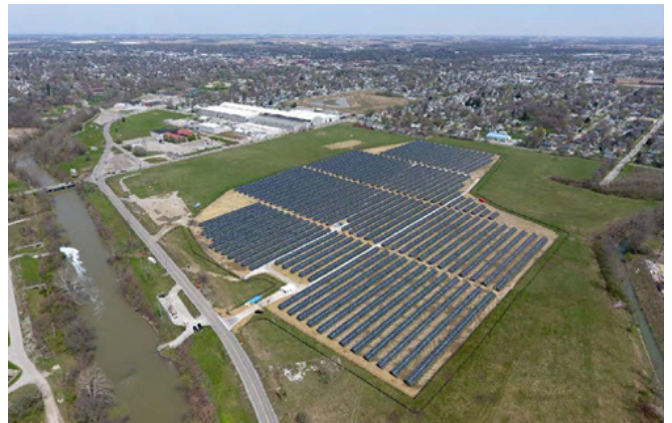
Onsite Solar Farm: Construction and operation plans for the 27-acre solar farm were designed to accommodate mowing and other routine activities needed to maintain the underlying soil cover. The solar panels are mounted to a single-axis tracking system, allowing them to follow the sun's path throughout the day. Adjacent space is available for potential expansion of the farm. (photo source: IDEM)
