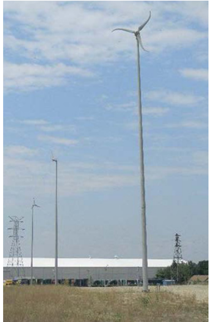
Onsite Wind Turbines: Three wind turbines operating in the former quarry area offset the use of grid electricity to extract contaminated groundwater.
