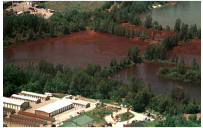
Former Acid Lagoons: The 56-acre acid lagoon area contained 10 lagoons that received spent pickling and finishing liquors from the main plant. Prior to remedy construction, the area's settling ponds were stabilized through acid neutralization. (photo source: Kokomo Tribune)
