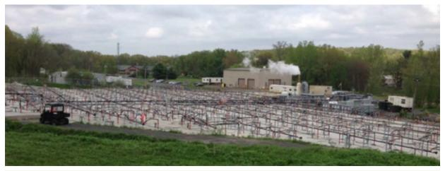
**ISTR Operation:** Thermal remediation was conducted in a 1.75-acre area in 2014-2015. The system employed more than 1,400 heaters, vapor recovery and monitoring wells. ISTR removed approximately 99.5% (nearly 500,000 pounds) of the soil's solvent contamination. *Image credit: SRSNE project website*
