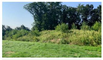
**Cap Vegetation:** The soil/sediment cap surface was seeded with native grasses requiring no irrigation. Routine maintenance includes yearly mowing, re-seeding any bare ground, and occasionally removing invasive vegetative species by way of herbicidal spot treatment.
