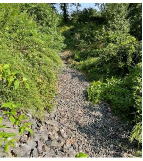
**Rock-Lined Channel:** Native plants line the sides of a rock-lined channel designed to carry stormwater to a downgradient, onsite discharge area. The vegetation helps prevent erosion while filtering the stormwater, promoting stormwater infiltration, and slowing the flow of additional stormwater entering the channel.
