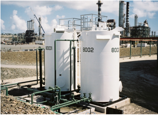
Recovered Product: Recovered subsurface fluid accumulates in aboveground tanks at the adjacent petroleum facility, where recovered oil is reclaimed for beneficial use.
