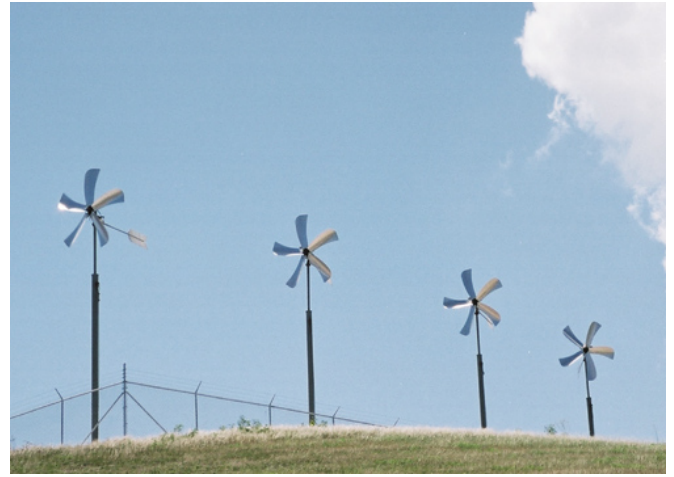
Wind Field: Prior to 2011, when this wind field was taken out of service, trade winds averaging 11 mph brought nearly a constant source of renewable energy for remediation at the Former St. Croix Alumina site.
