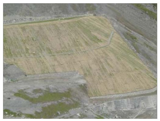
Reprofiled dam with improved drainage, reduced gradient and stabilised walling. Note the grass growth through matting, mid-slope stone drain and sheep!!! Note also the two new retaining walls at the toe of the dam.
