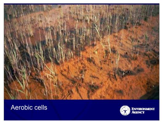
Significant deposition of ochre (Fe(III) oxyhydroxides) at front of first aerobic cell (80-98% of Fe(II) oxidised). Photo June 2002.
