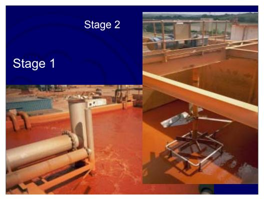
Stage 1 reactor. Addition of minewater (large pipe - pH~3.5) AND recirculated sludge to neutralise (pH 6-8) and precipitate (oxy)hydroxides. Sufficient agitation to keep precipitates in suspension - retention time 30 minutes.
