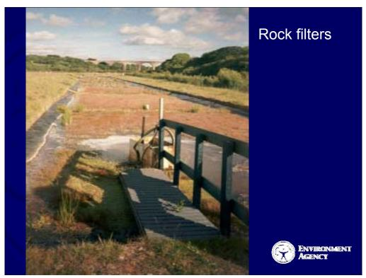
Rock filters - algae-colonised shallow rock pools relying on oxygenic photosynthesis to locally raise the pH to precipitate Mn. pH was typically 5-6, too low for Mn precipitation.
