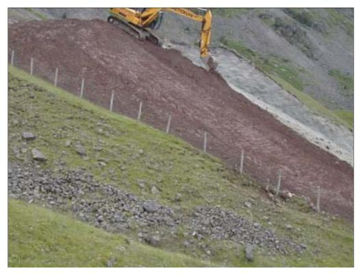
Gradient reduction, exposure of tailings kept to a minimum by progressive application of soil cover. The crest of the slope was cut back and in places increased in height to improve the fall back to the drain behind the dam.
