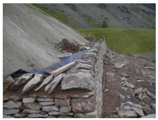
Reducing the gradient - local construction of stone-filled gabion baskets on concrete foundations with stone-faced walls. As Scheduled Ancient Monument, archaeological investigations were needed before walling could start.
