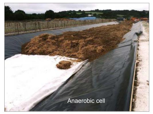
Anaerobic reactor - geomembrane-lined cell filed with mixture of straw, sawdust and manure - long and short-term source of organic carbon. Limestone was also added to the untreated source to add alkalinity.
