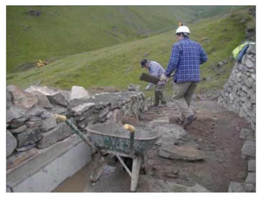
A stone-filled French drain was installed locally through scree behind an area of elevated water level in the dam to intercept and discharge shallow groundwater flow through the scree. The surface drain at the back of the dam was widened and deepened to capture surface water run-off and shallow (<1m) groundwater from the screes. The width of the drain was overdesigned to permit easy access for maintenance.
