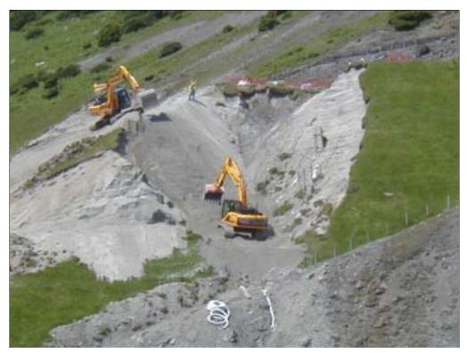
Cutting back the gradient and fill of the failure void with coarse to medium sand tailings in compacted layers, progressively loading the toe and improving the stability of the failure scar.
