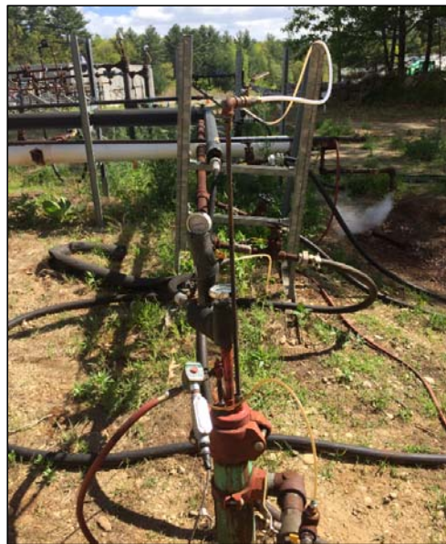
Well with both slurping and pneumatic pumps installed
