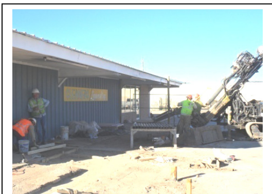
Figure 4. Angle Drilling.
