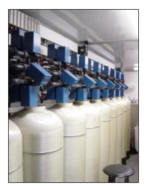
Photograph 2: Interior of Basin Water high efficiency ion exchange system.
