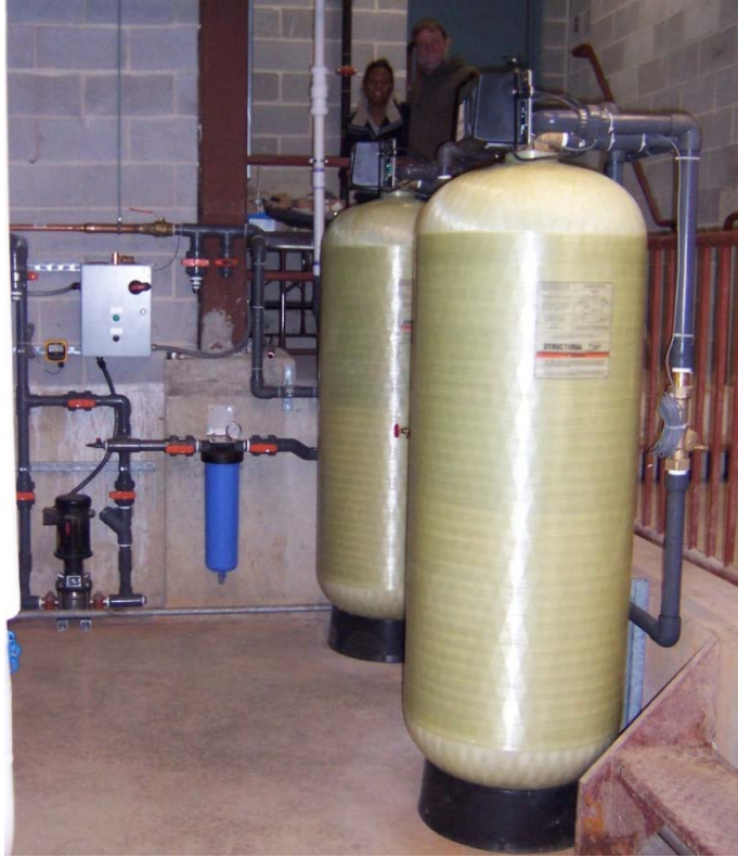
Figure 2-1A. 20-gpm Adsorbisia™ GTO™ Media System by Siemens (Two FRP Vessels in Series)
