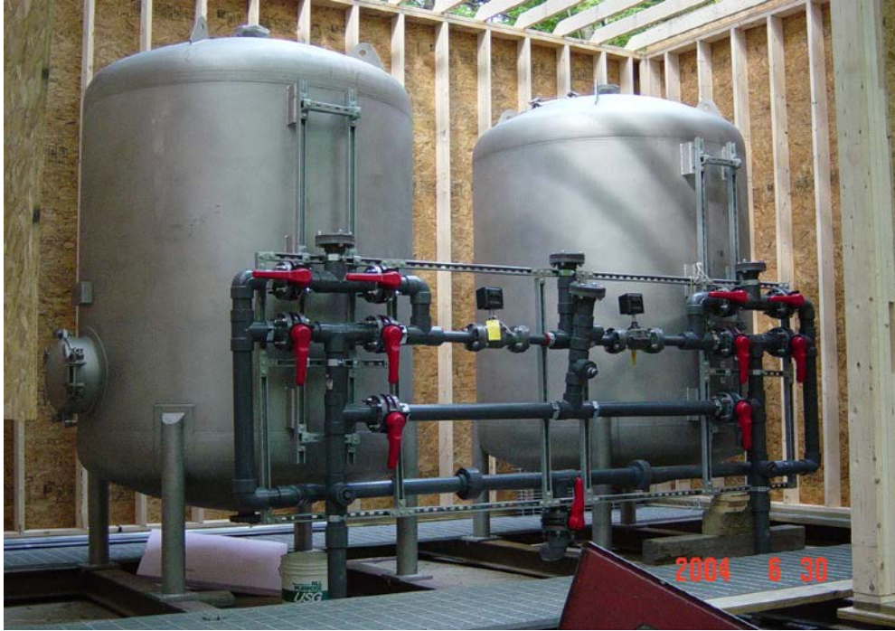
Figure 2-1C. 40-gpm G2 ® Media Arsenic Adsorption System by ADI (Two Stainless Steel Vessels in Series)
