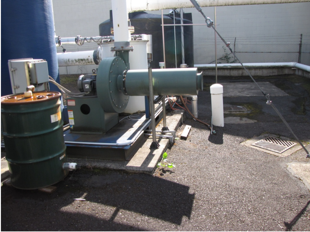
Photo 3. Liquid carbon treatment drum and secondary containment (catch basin effluent routed through VOC treatment stream).
