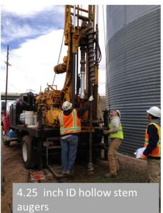
Figure 3-5. Central Mining Equipment (CME) hollow-stem auger (HSA) drilling system
