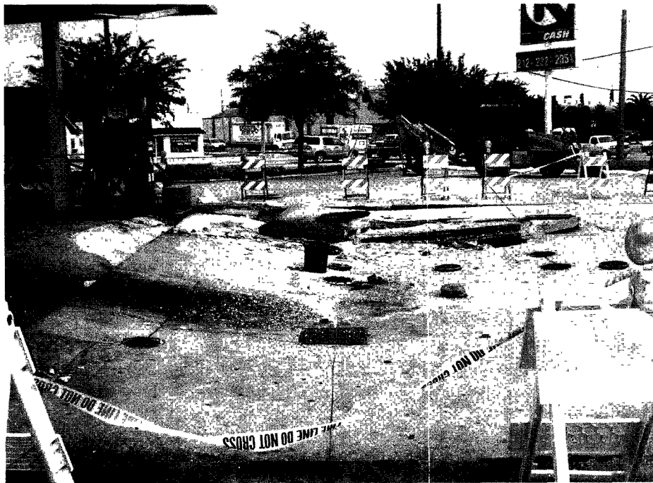
The lightning-impacted site showing subsidence of the tank pad over the UST area.
