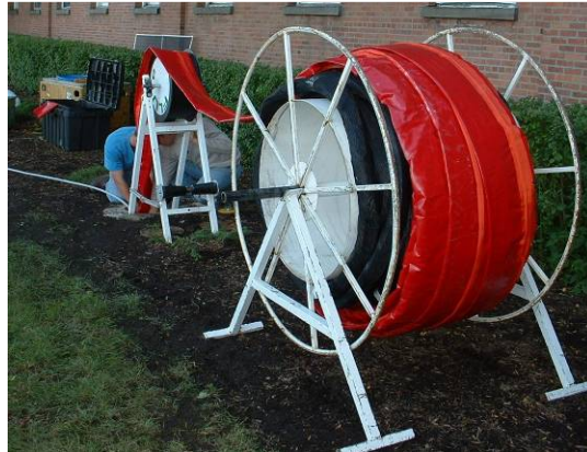
Figure 3-2. Water FLUTE™ Installation at the Watervliet Arsenal
