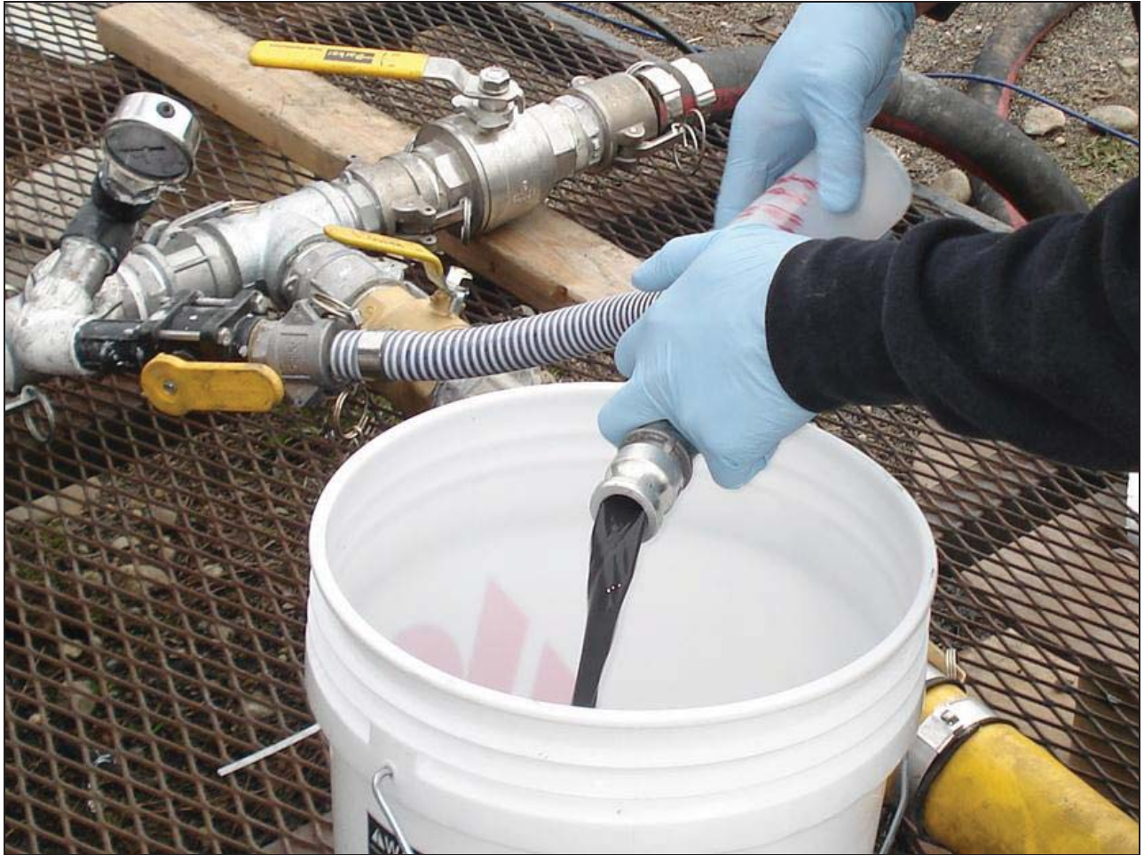
Figure 5-18. Picture of ZVI injection solution during injection.
