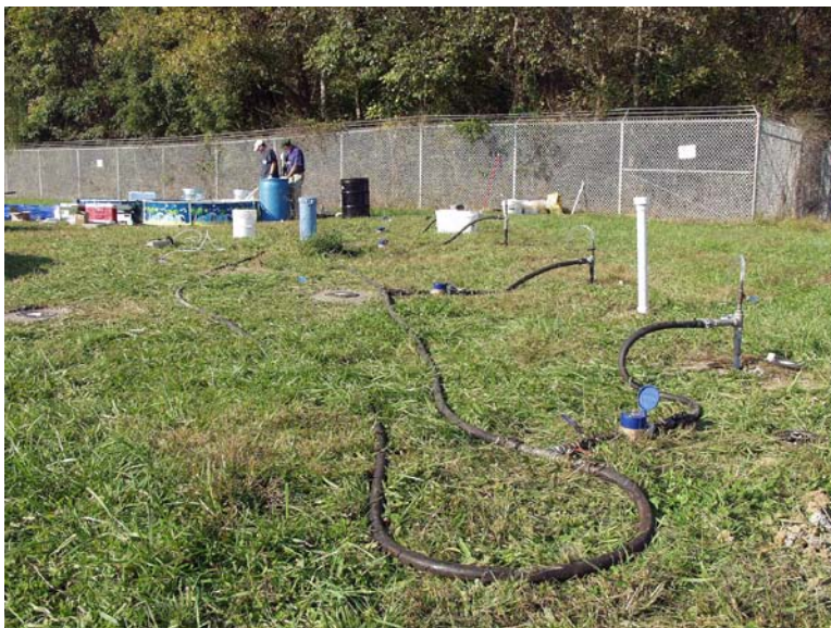
Figure 3. Injection of EOS ® to form the permeable reactive barrier.
