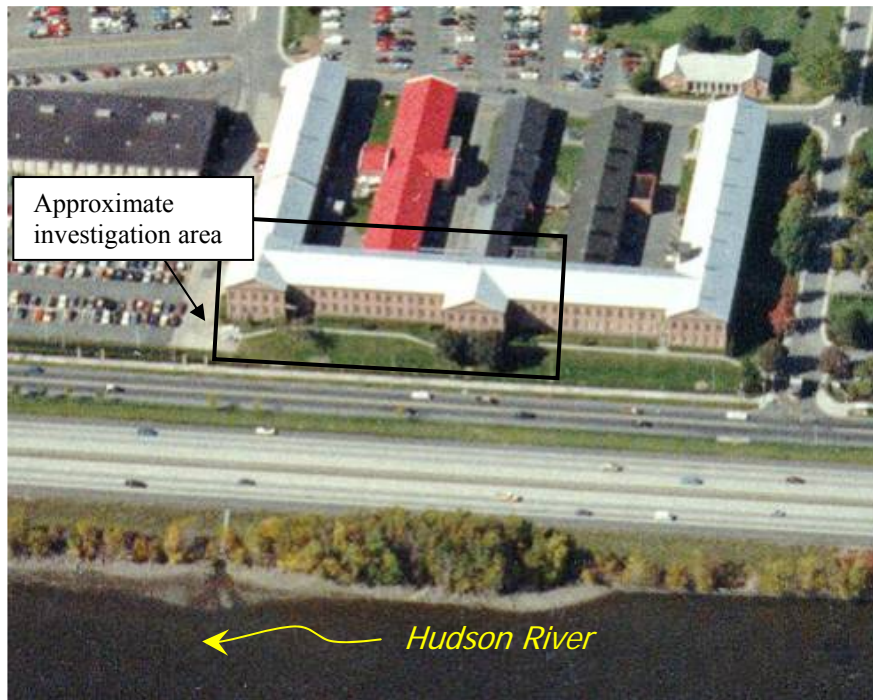
Figure 1-1: Building 40, Watervliet Arsenal
