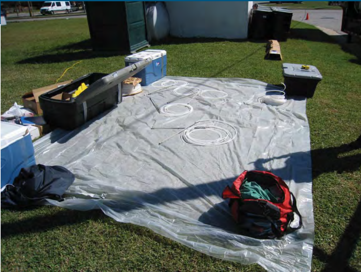
Photo 9. Preparation and staging of materials used in the installation of the micro-wells.
