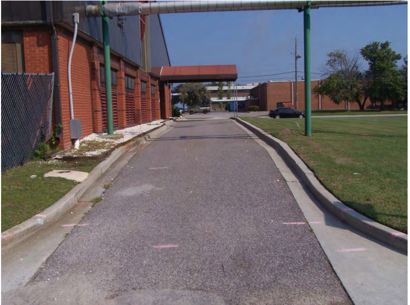
Photo 4. Looking north from the southeast corner of the new Dry Cleaner building and laundry pick-up drive-through. The source area of the plume is the general area in the southeast corner of the building (left side of drive-through).
