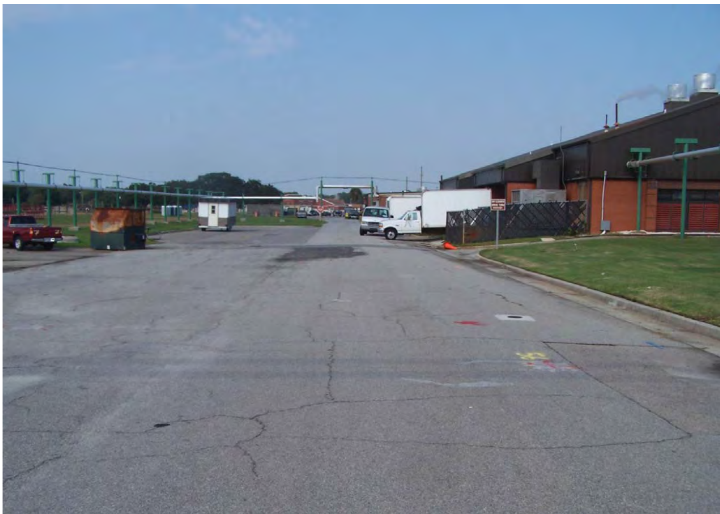
Photo 2. Site 45 looking west from the middle of Kyushu Street, and the new Dry Cleaner building (Bldg 192) is on the right.
