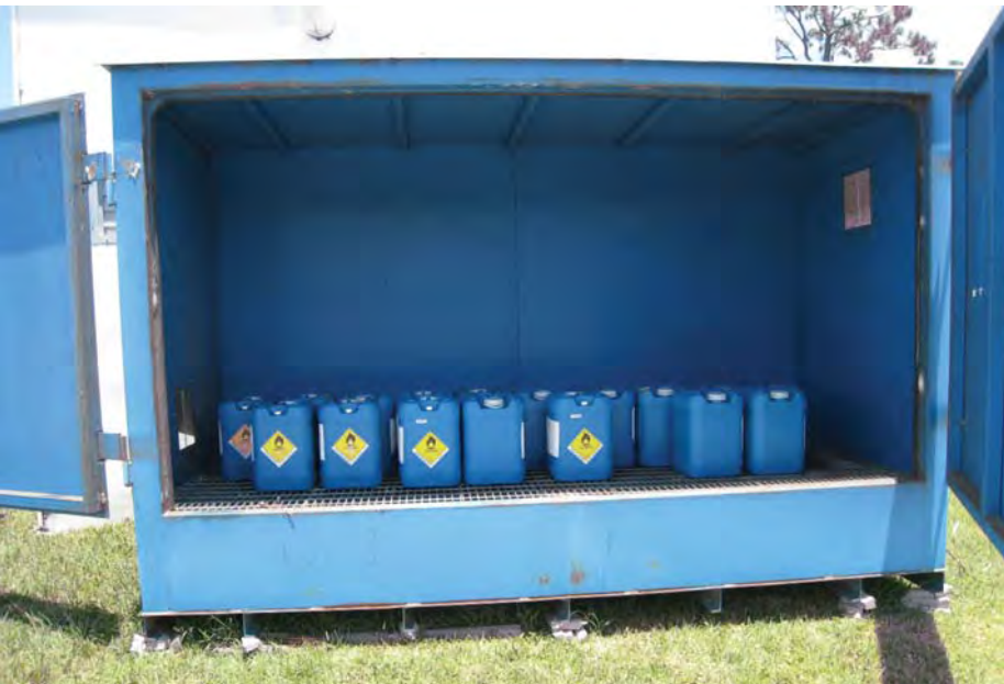
Photo 18. Storage of 5 gal pails (jerricans) of 40% liquid sodium permanganate in the hazardous waste storage and containment unit.
