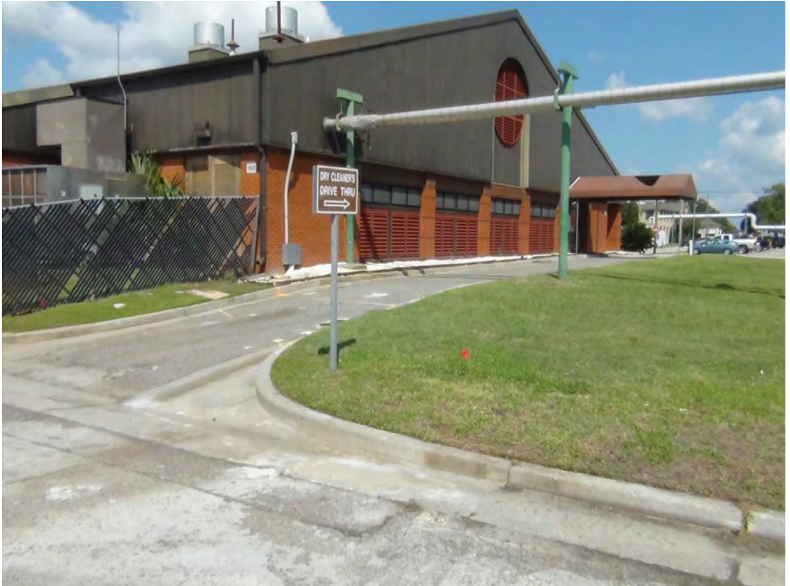
Photo 3. Site 45 looking upgradient from the middle of Kyushu Street towards the new Dry Cleaner building. The approximate centerline of the plume is from the near corner of the dry cleaner building and extends in the southeastern direction.
