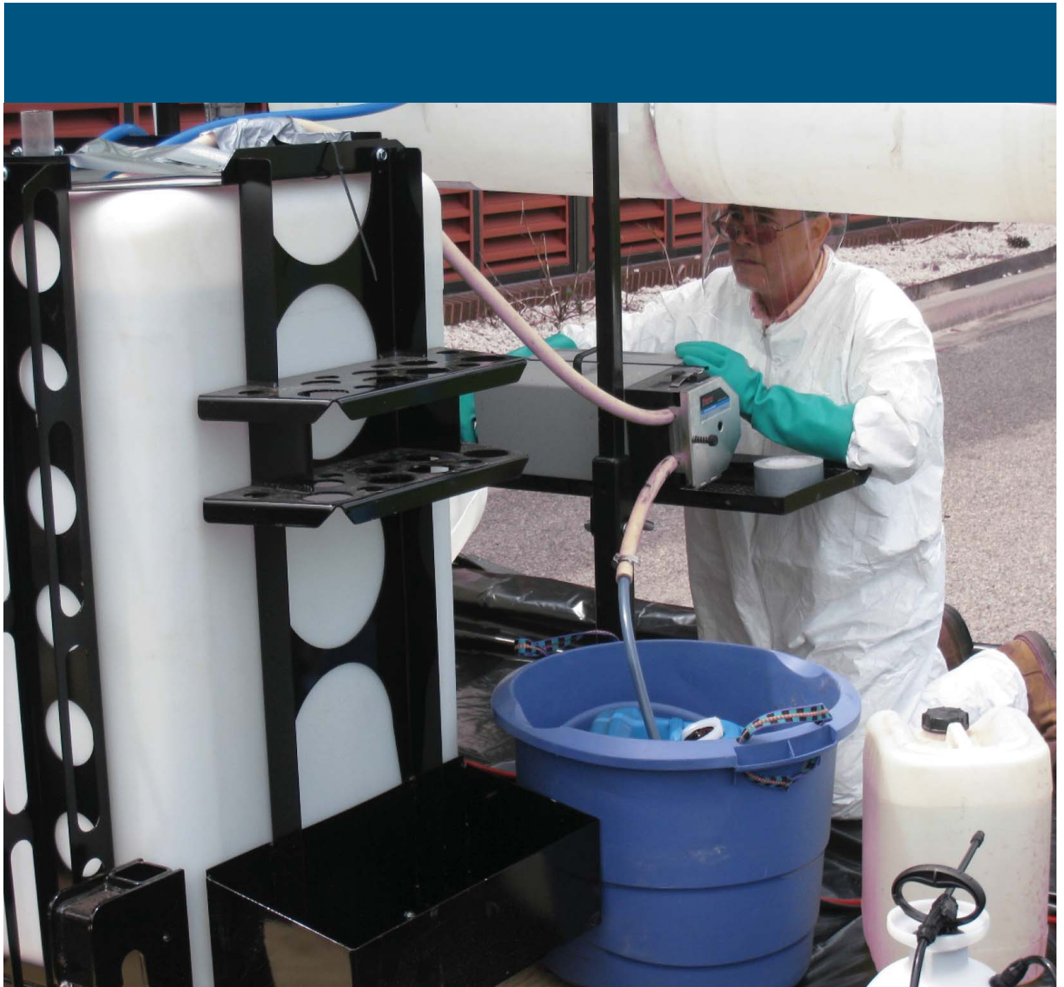
Photo 24. Using a peristaltic pump to transfer a specific volume of 40% liquid sodium permanganate into the mixing tank. Water was introduced into the mixing tank at high flow rates to assure mixing of the sodium permanganate and to achieve the targeted oxidant solution concentration needed for injection. A secondary containment system was constructed under the oxidant injection system.
