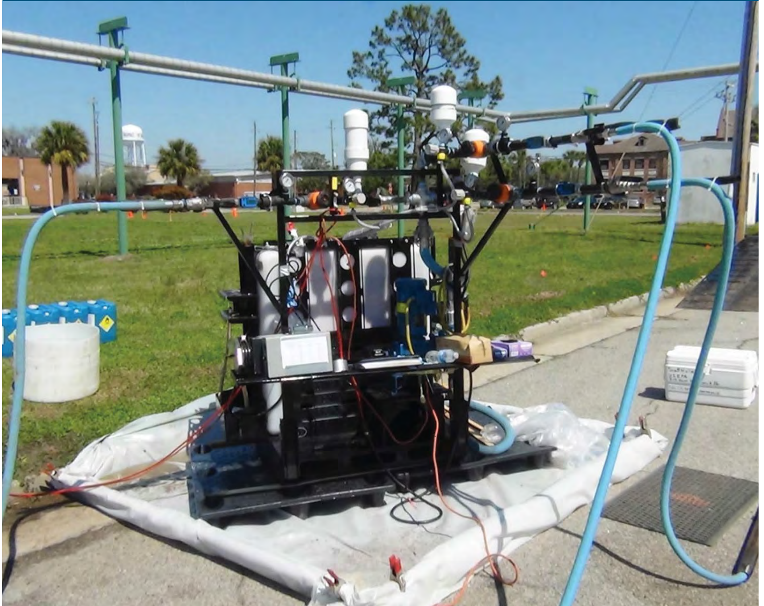
Photo 23. The oxidant injection system delivering oxidant to 3 injection locations.
