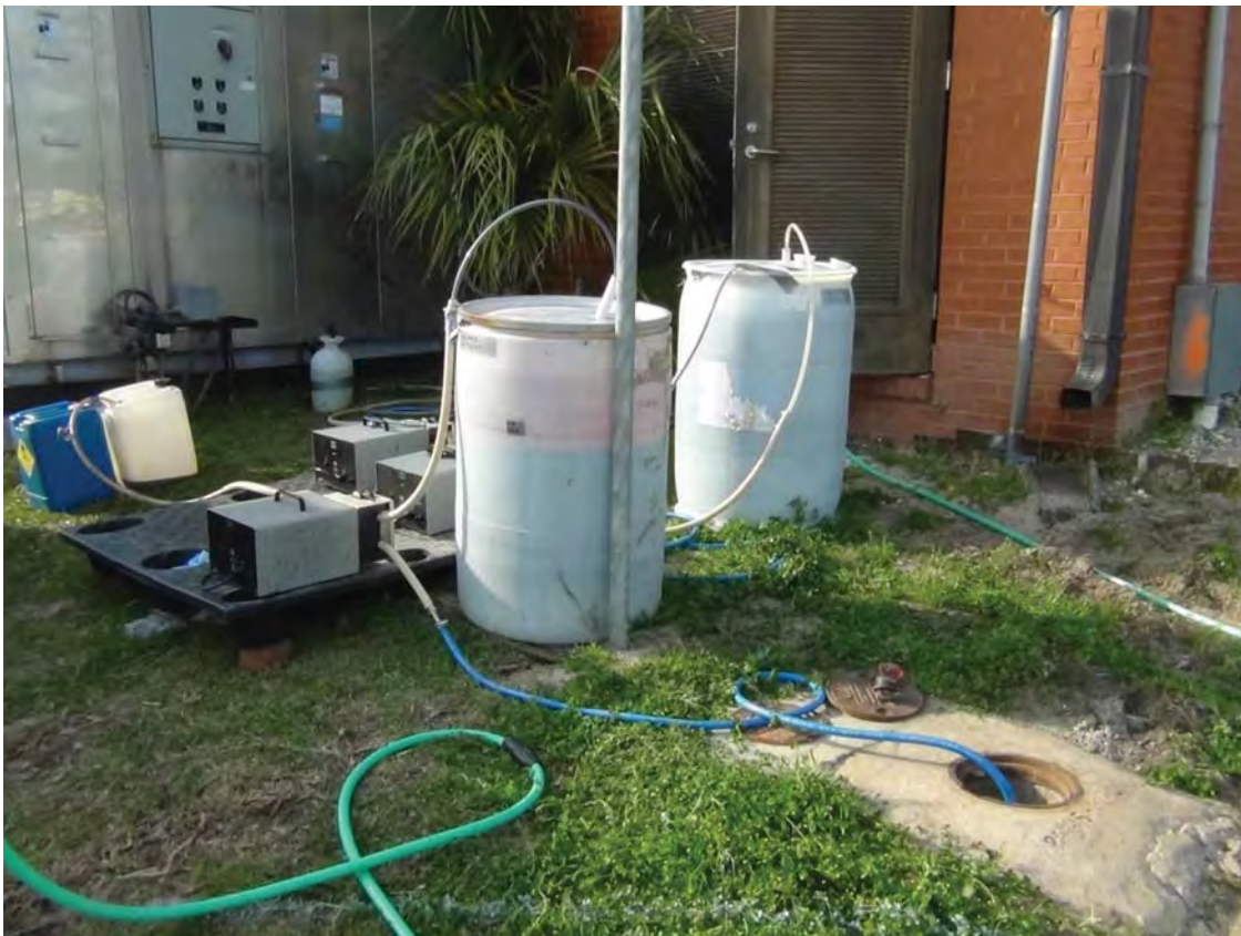
Photos 31-32. Pumping oxidant into well MW-25 and Inj. 1-Deep at approximately 2-4% \text{NaMnO}_4 .
