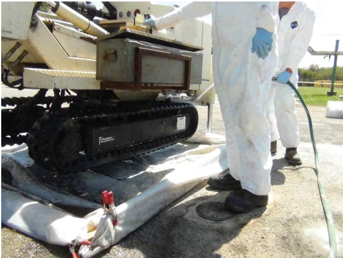
Photo 33-34. Decontamination of GeoProbe rig prior to departure; capture of investigation derived wastewater for subsequent testing and disposal.
