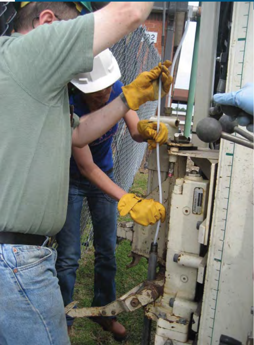
Photos 12-13. Closeup of the installation of the micro-well well screen and tubing through the Geoprobe rod. The Geoprobe rod and tubing is filled with water to prevent heaving and sand-binding of the tubing inside the rod. The tubing and screen are held in place as the Geoprobe rod is retrieved.
