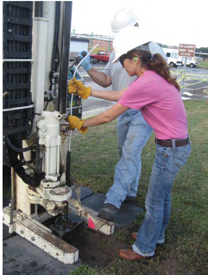
Photos 12-13. Closeup of the installation of the micro-well well screen and tubing through the Geoprobe rod. The Geoprobe rod and tubing is filled with water to prevent heaving and sand-binding of the tubing inside the rod. The tubing and screen are held in place as the Geoprobe rod is retrieved.
