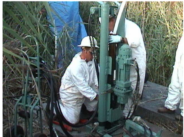
Figure 19. Preparation and installation of Multilevel Monitoring System (MLMS) at wetland study site: (clockwise from upper left) coiled 7-chamber polyethylene tubing, preparation of MLMS with sand packers and bentonite packers, drilling of borehole with vibratory rig, and insertion of MLMS down borehole casing. Precision Sampling, Inc. photos
