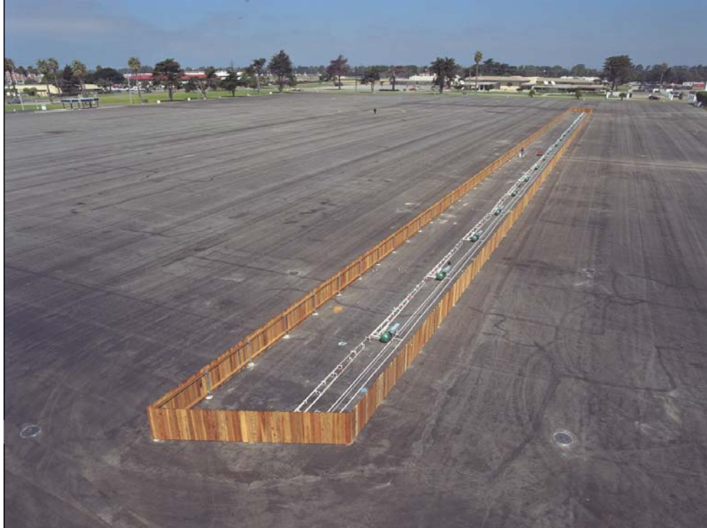
Figure 3. Large-Scale Biobarrier PTB System at NBVC. (The fenced-in area is approximately 600-ft long.)
