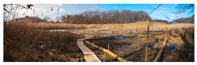
Figure 7. Cleared test plots, staked sediment control products, and temporary walkways.
