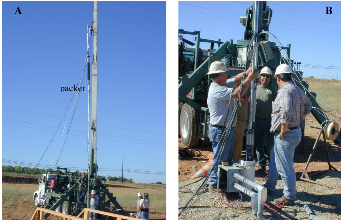
Figure 2.2. Photograph of Equipment Installation into the Downflow HFTW at Aerojet. The packer is visible in panel A and the wiring, tubing, and equipment present in the HFTW is seen in Panel B.
