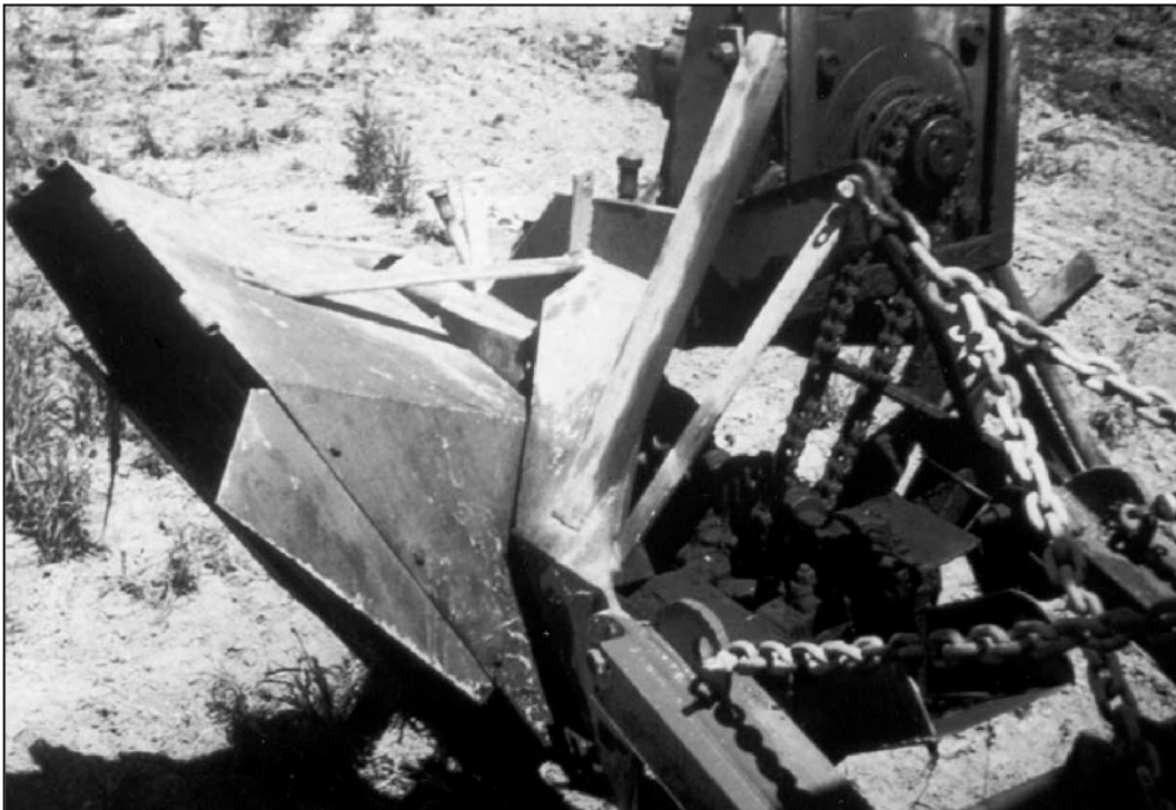
Figure 4-40. Trapezoidal Rotary Trenching Implement
