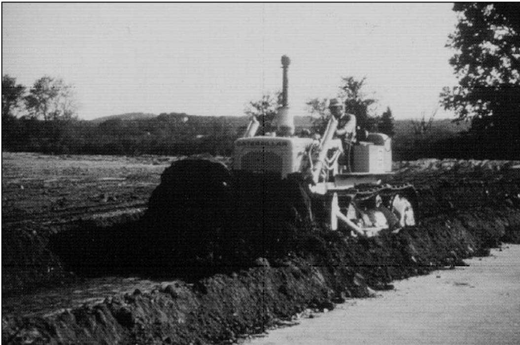
Figure 5-27. Liming and Mixing Layers of Silty and Sandy Dredged Material at Nott Island Upland Site, Connecticut River, CT, in the 1970s; This Site has been a Nesting Meadow and Songbird Habitat for More than 25 Years
