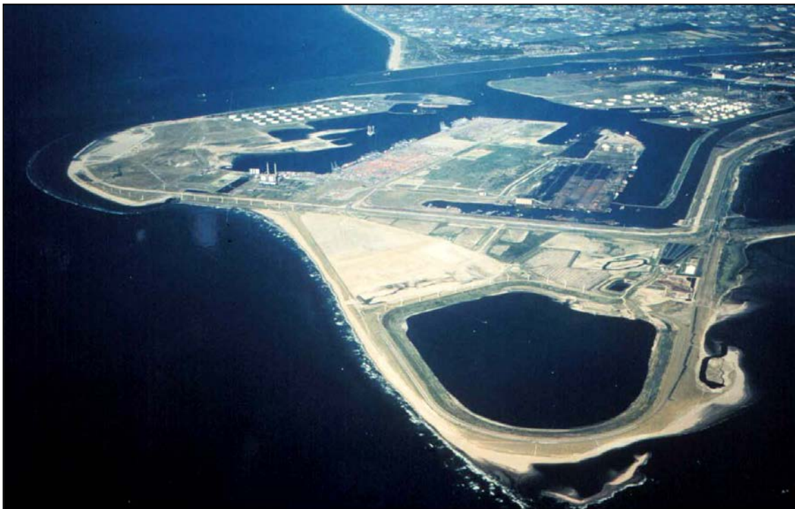
Figure 4-2. Shelfter CDF in Rotterdam, The Netherlands
