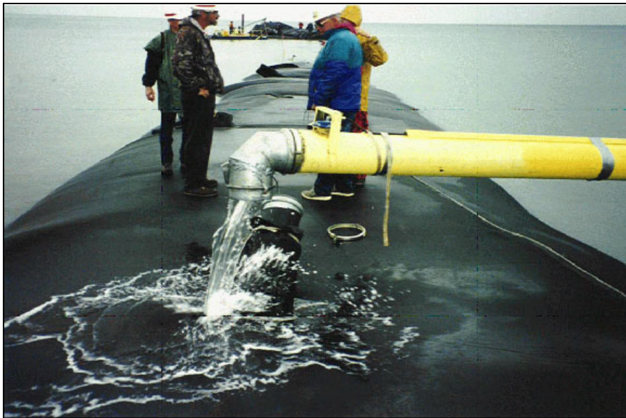
b. Filling a Custom-Designed Geotextile Tube with Dredged Material in Chesapeake Bay, MD, for Erosion Control and Sediment Stabilization
