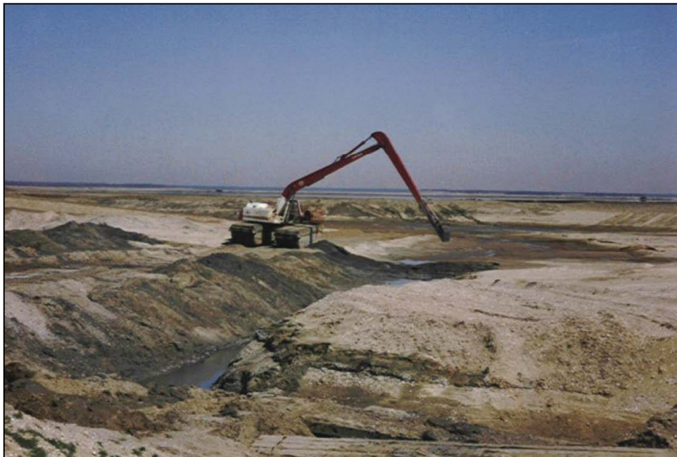
b. Trenching the North Cell of Dredged Material on Hart-Miller Island to Maximize Dewatering, so the Site can be Filled to Capacity prior to Wildlife Habitat Development
