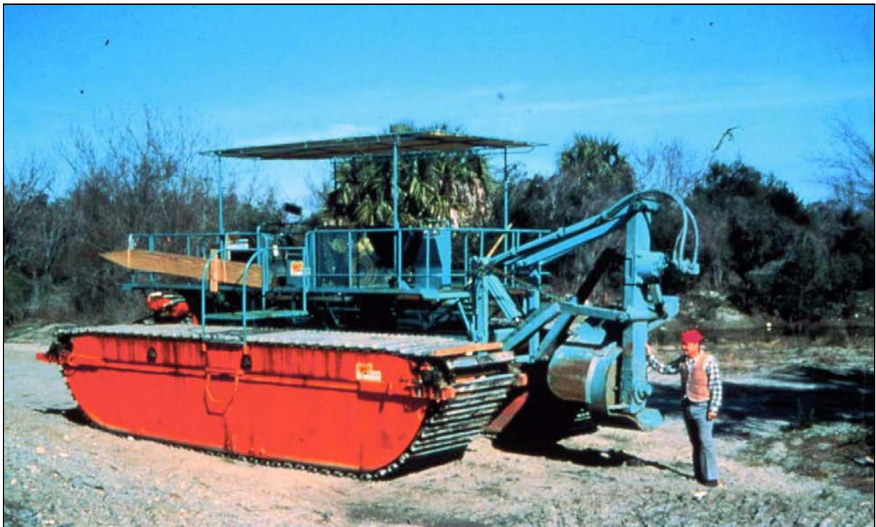
Figure 4-38. Track-Mounted Rotary Trencher Used in Mosquito-Control Activities
