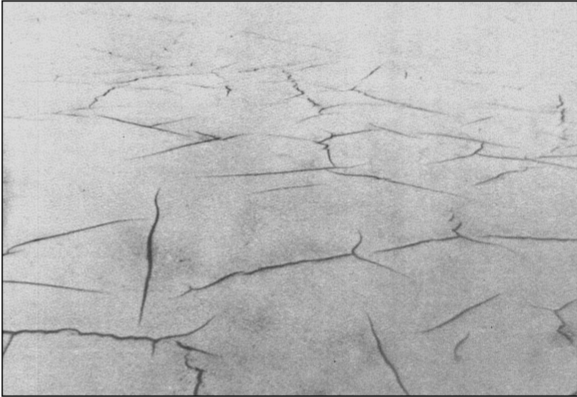
Figure 4-30. Surface of Fine-Grained Dredged Material at the Earliest Time when Surface Trenching Should be Attempted
