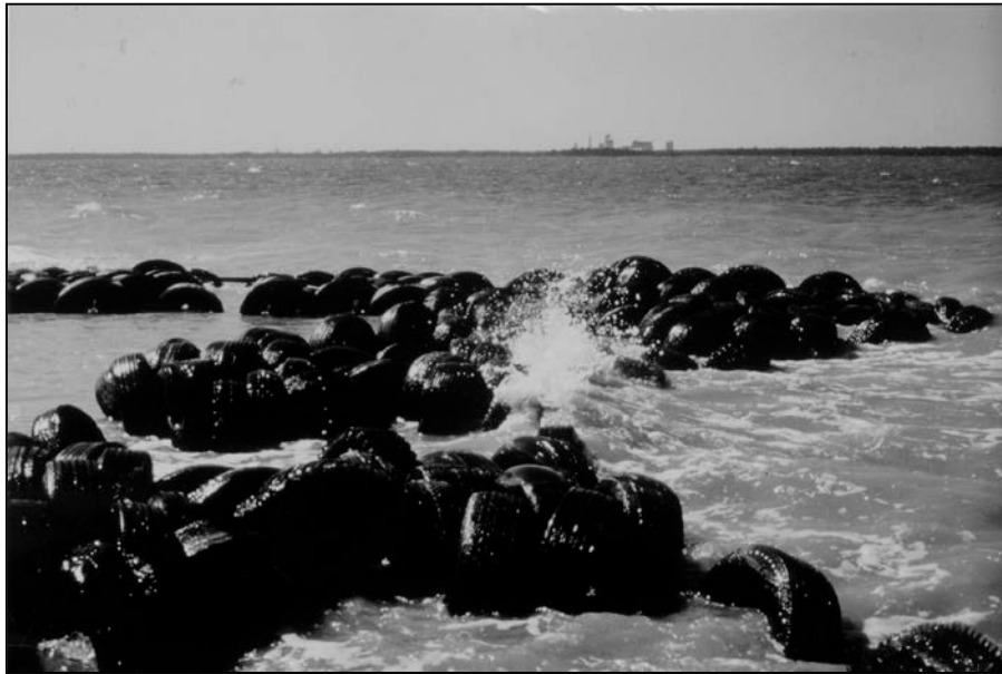
a. A Floating Tire Breakwater Installed at Gaillard Island, AL, to Protect Newly Planted Marsh from Moderate Water Energies; Floating Breakwaters must be Prevented from Breaking Loose into Open Water
