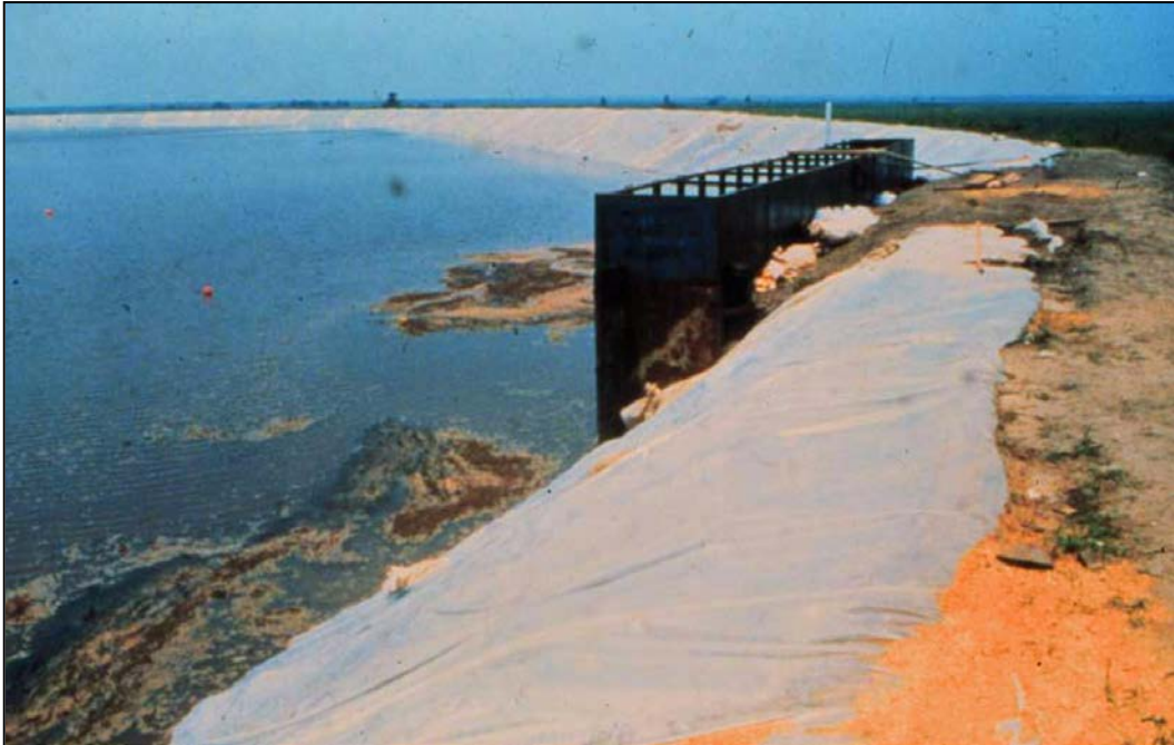
Figure 4-19. Rectangular Weir (1)
