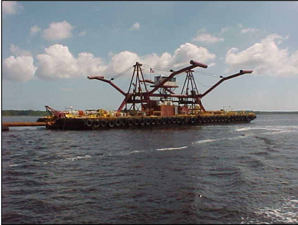
Figure 2-27. Spider Barge Connected to a Hydraulic Pipeline Dredge
