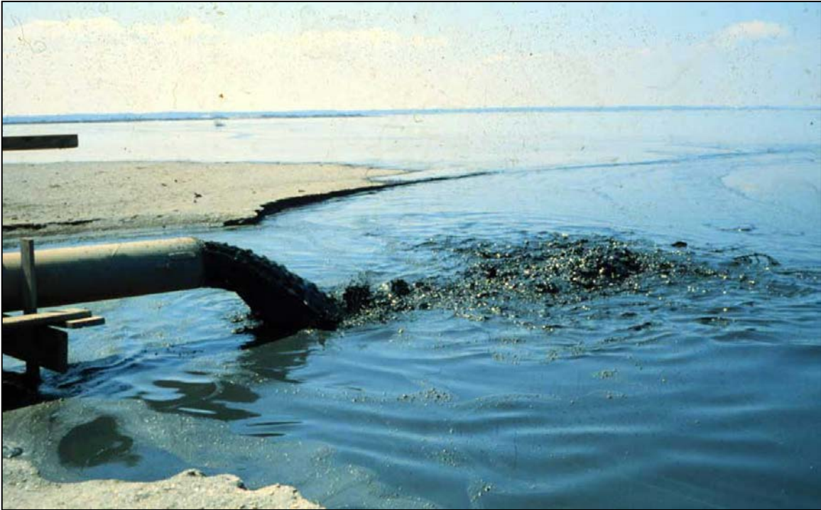
Figure 4-6. Typical CDF Hydraulic Inflow from a Cutterhead Pipeline Dredge
