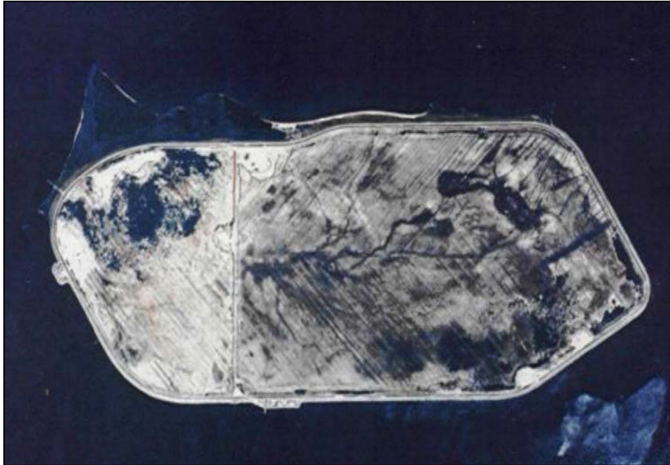
a. An Aerial View of the North and South Cells of Hart-Miller Island, which Consists of 445 ha of Dredged Material and which will be a Recreation/Wildlife Habitat Site when it is Completed; Note the Dewatering Trenching Lines in both Cells
