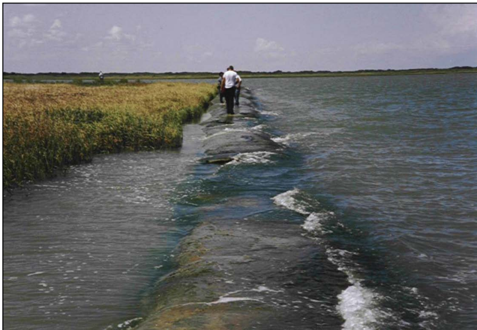
b. Dredged Material-Filled Geotextile Tubes Fronting the Planted Saltmarsh at Aransas National Wildlife Refuge
