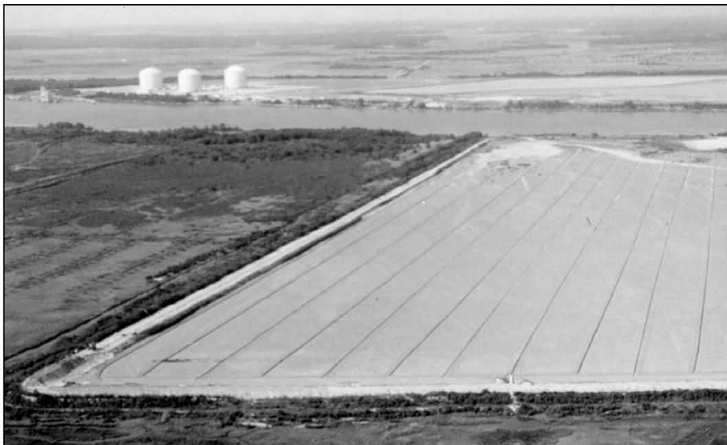
Figure 4-44. General View of a Confined Disposal Area Showing Parallel Trenches in Place
