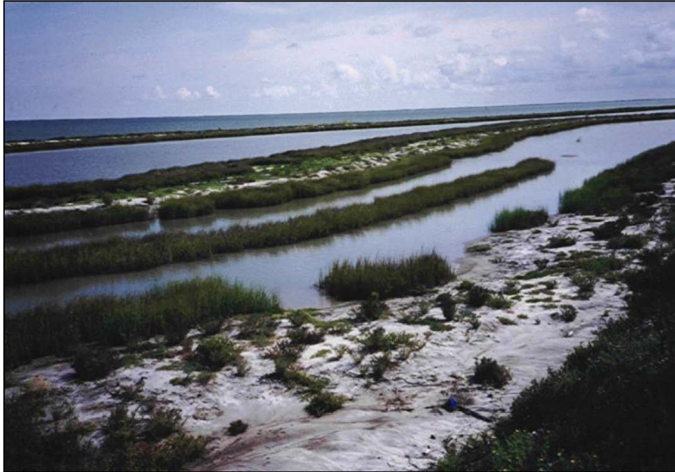
a. Saltmarsh Restoration Using Dredged Material and Bioengineering Structures at Aransas National Wildlife Refuge in 1994; the Site is less than 6 Months Old in the Photograph
