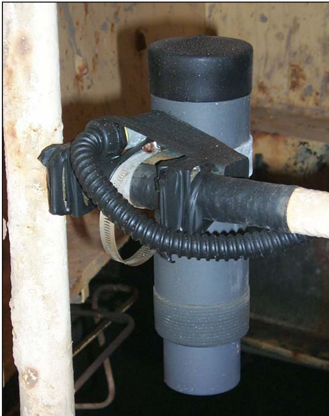
Figure 2-45. Acoustic Hopper Level Sensor
