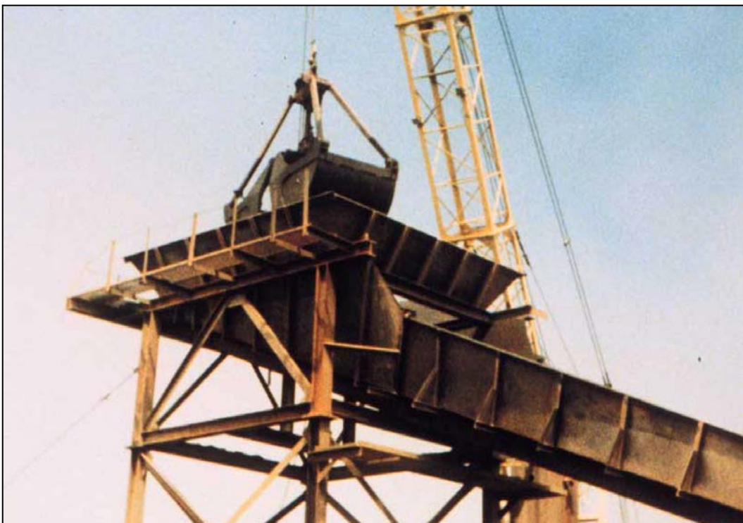
Figure 4-9. Chute Used for Direct Mechanical Placement into a CDF
