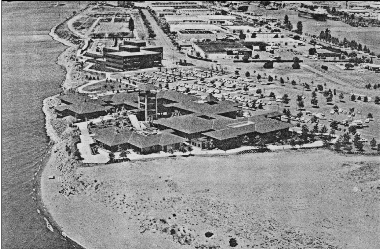
Figure 5-69. A Large Shopping Mall, Port Center, which was Built on Dredged Material at Swan Island on the Columbia River at Portland, OR, Includes Shopping and Commercial Areas as well as Low-Rise Office Buildings
