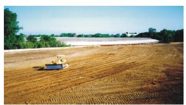
Regrading of the disturbed portion of the low-lying area following remediation. View is looking north towards the permanent sheetpile dam and the Ottawa River.
