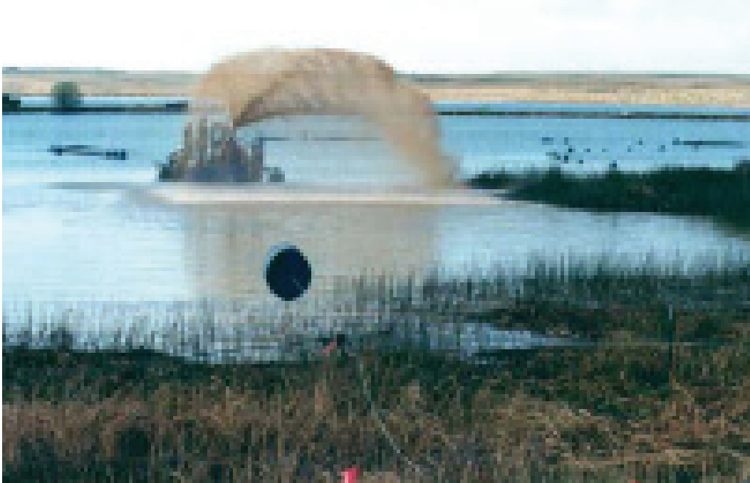
Figure 10. Sprayed slurry system placing sand at Soda Lake, Wyoming
