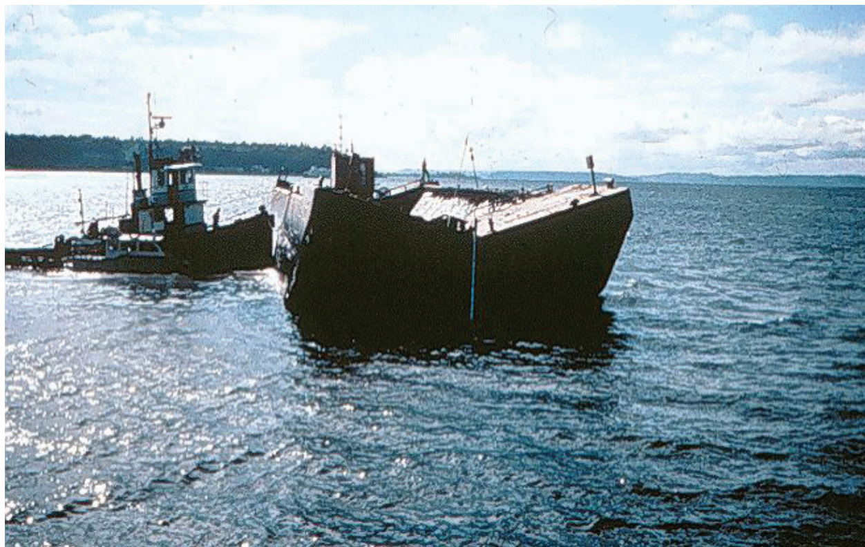
Figure 6. Spreading techniques for capping by barge movement at Denny Way, Puget Sound
