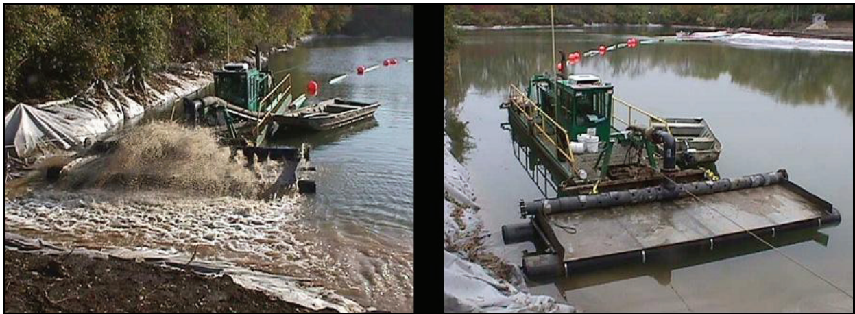
Figure 12. Spreader barge at Mock's Pond, Indiana
