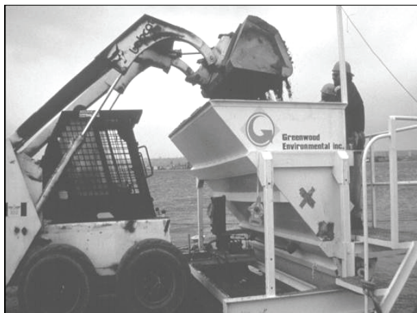
Figure 17. Tremie system employed at Hamilton Harbor, Lake Ontario
