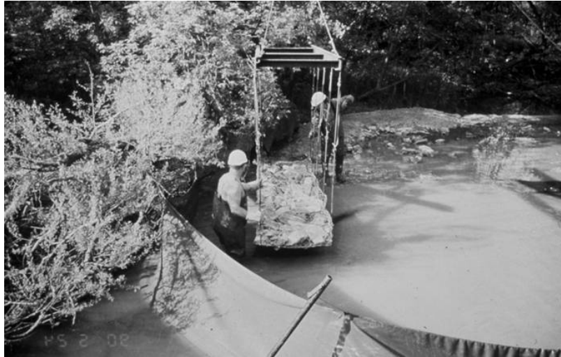
Figure 18. Stone placement at Sheboygan River
