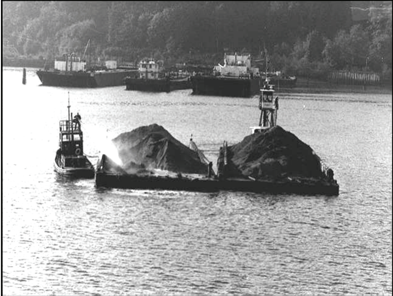
Figure 7. Hydraulic washing of coarse sand, Eagle Harbor, Puget Sound
