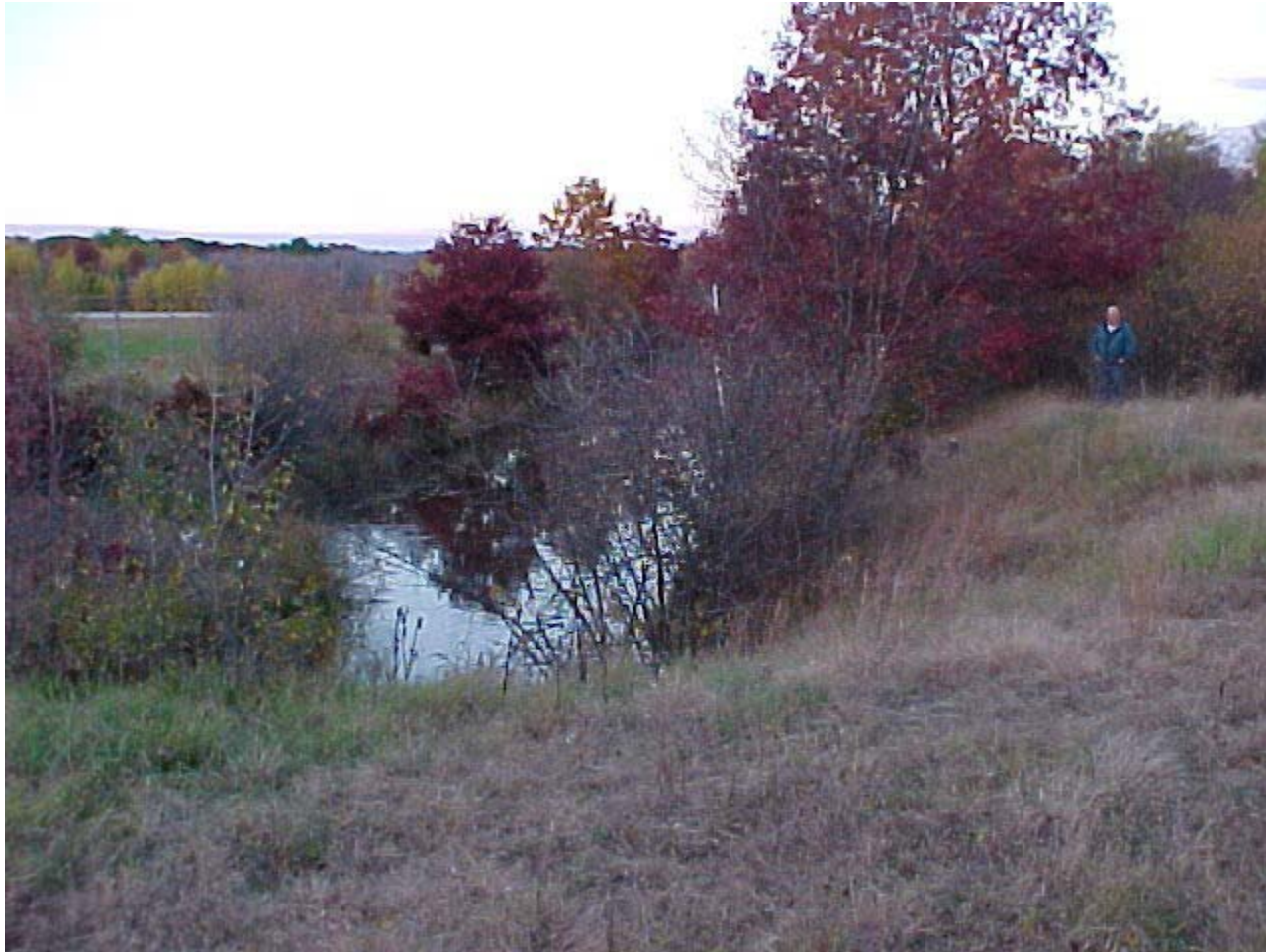
Figure 3-7. Drainage Channel Looking Northeast
