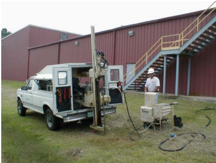
Figure 5.4 Pure Edible Oil Injection through Geoprobe® Rods Using a Grout Pump
