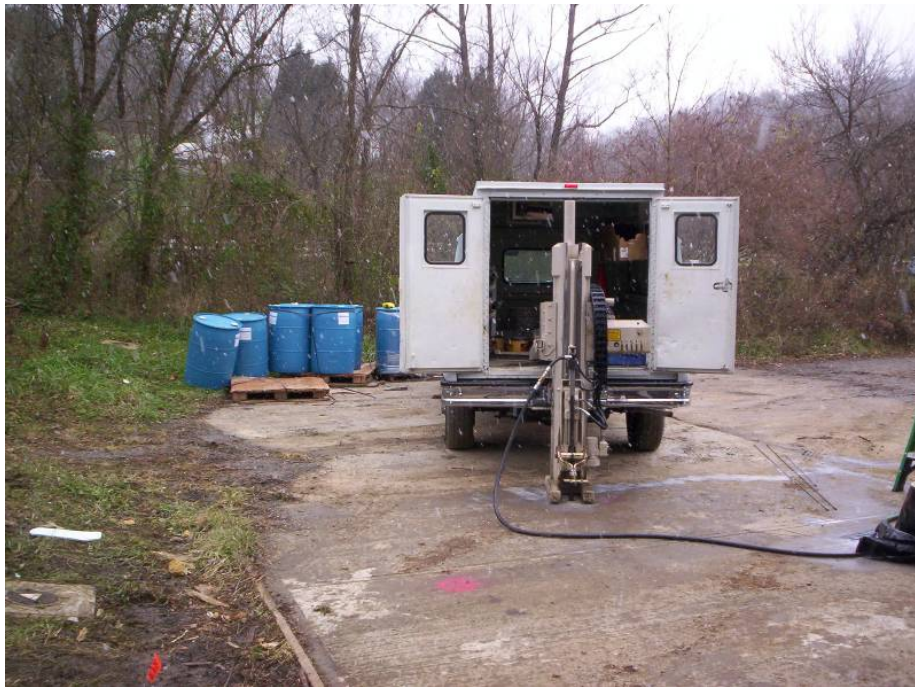
Figure 10. Direct Injection Using a Geoprobe® for Full-Scale Injection
