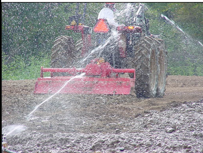
Application of DARAMEND® at the T.H. Agricultural and Nutrition Superfund Site (Source: Adventus Americas, Inc.).
