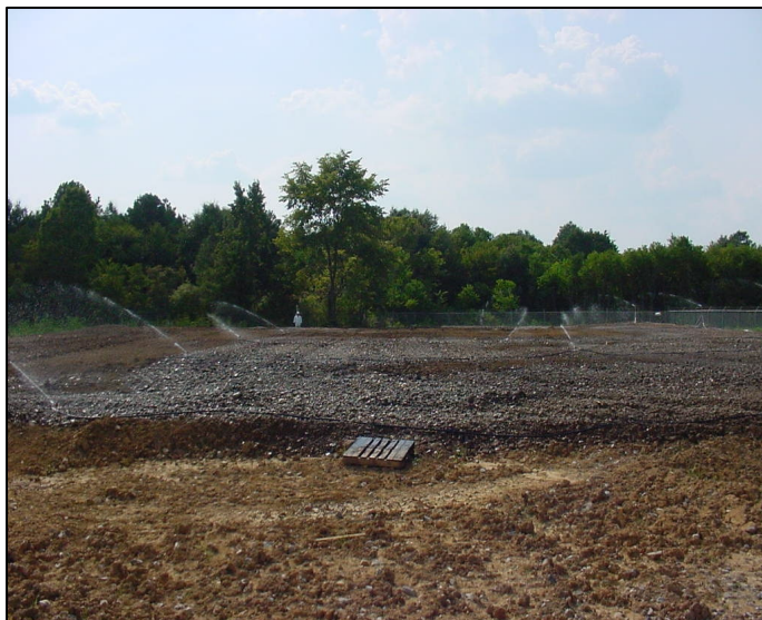
Bioremediation using DARAMEND ® process. Ref. 1
