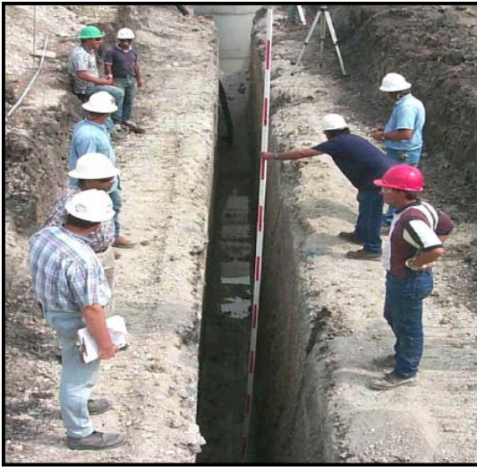
Figure 7. Continous PRB Trench Excavated to Add Solid Substrate. (Reprinted from DNEP, 2001)
