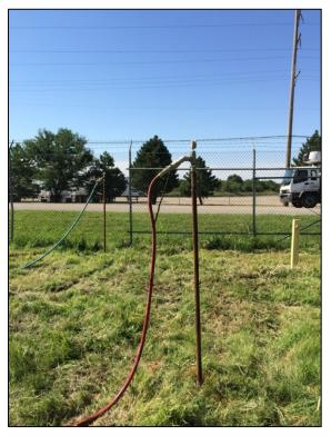
Photo 12: EHC injection rod with hose connected to injection manifold.
