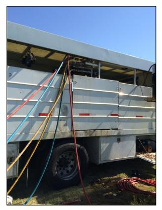
Photo 13: Hoses connected to injection manifold in trailer.
