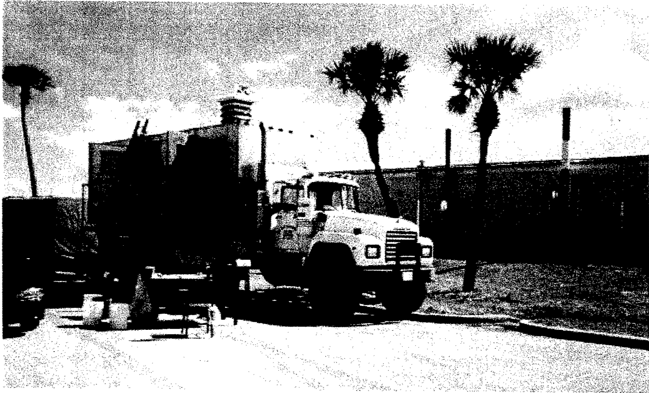
Figure 4-4. Outdoor Cone Penetrometer Test Rig for Soil Coring at Launch Complex 34
