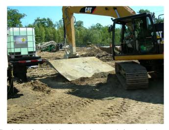
Steel plate found in the excavation; now being used to minimize rutting near the soil mix truck
