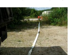
Water line installed from fire hydrant to mixing area
