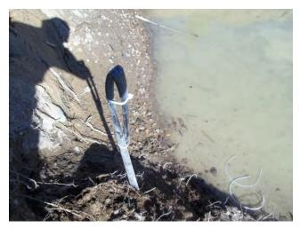
Duct taped and crimped black poly line water line to prevent sediment from entering EW-13B
