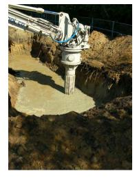
Soil mixing in cell E17 S15 (notice bubbling from chemical reaction)
