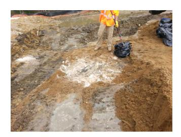
Containerizing the hydraulic fluid and associated impacted soil.
