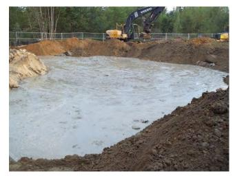
Swelled material to original grade in test cell.
