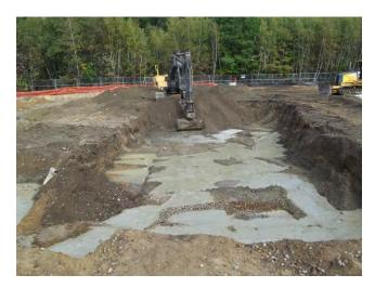
Excavating the relief cell for the swelled material located south of the soil mixing excavation.
