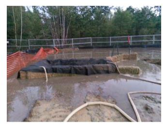
Hay bale and geotextile structure to filter water pumped from the excavation.
