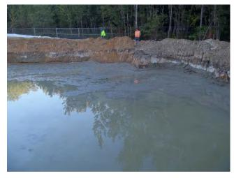
Removing the silt fence prior to re-establishing the access road on the eastern edge of the site.
