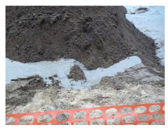
Swelled material exiting test cell over the temporary berm into the remaining portion of the exaction as the test cell is backfilled.
