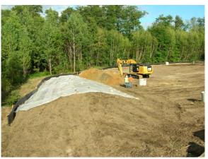
Topsoil stockpile partially covered and excavating overburden material in preparation for soil mixing on Monday
