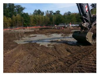
Attempt to blend soil mixing material with common fill. Very time consuming. Soil mixing material did not dry out after 1.5 hours and did not blend well when pushed with the bulldozer.
