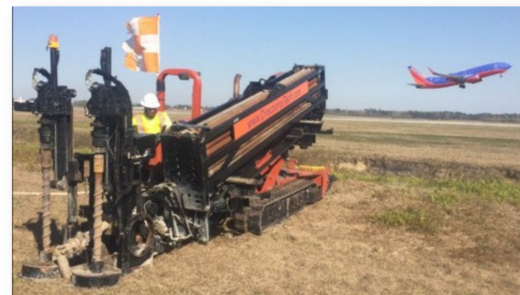
HDD installation of a biospargewell at Joint Base Charleston (DTI 2019)
