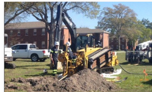
HDD installation of conveyance lines (Jacobs 2022)
