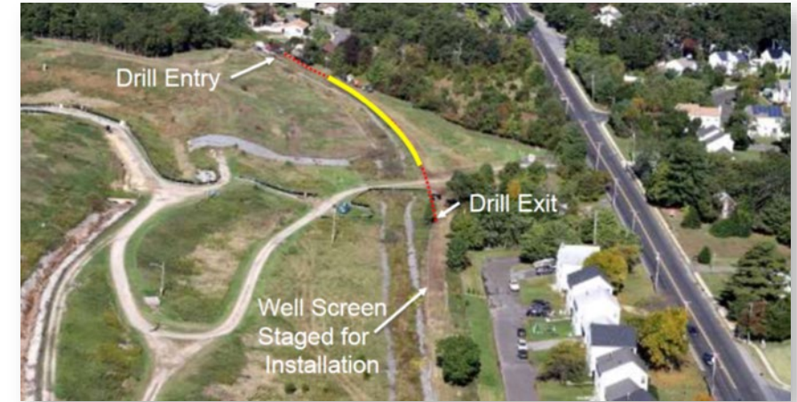
Horizontal GW extraction: aerial drone view (DTI 2016)
