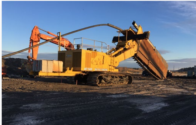
50-foot one-pass trenching (Geosyntec 2020)
