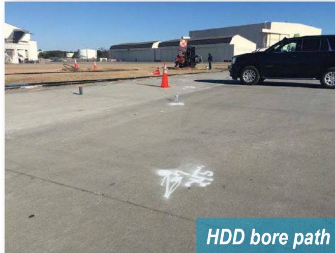
Horizontal biosparge well installation (FPM Remediations 2018)
