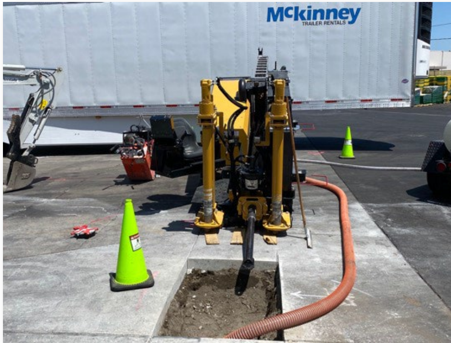
HSVE well installation (Geosyntec and EDTD 2021)
