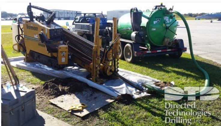
HDD for installation of horizontal air-spargewell installation at Eglin AFB (EDTD 2023)
