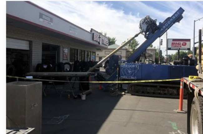
Angled sonic drilling (Gregory Drilling 2023)
