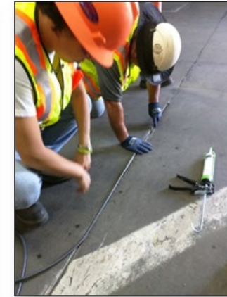
Joint sealing with flexible self-leveling silicone joint sealant (NOREAS 2018)
