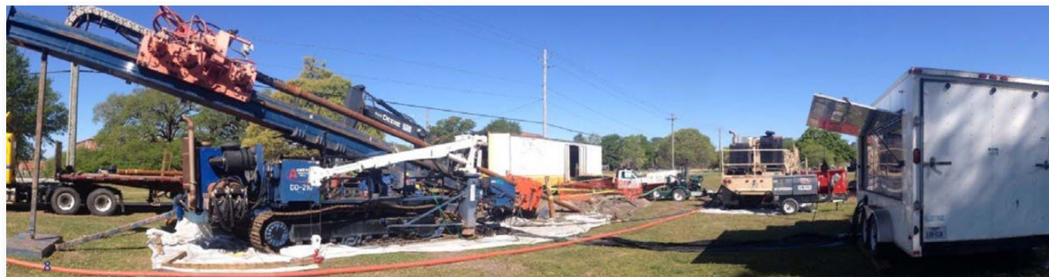
Pilot test horizontal injection well HDD installation and bit exit (Jacobs 2018)
