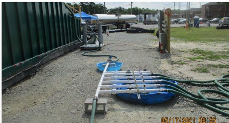
ISCO injection manifold and circulation equipment (Agviq 2022)
