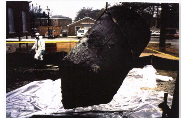
Past site remedial actions: UST removal (five USTs total) (Jacobs 2018)
