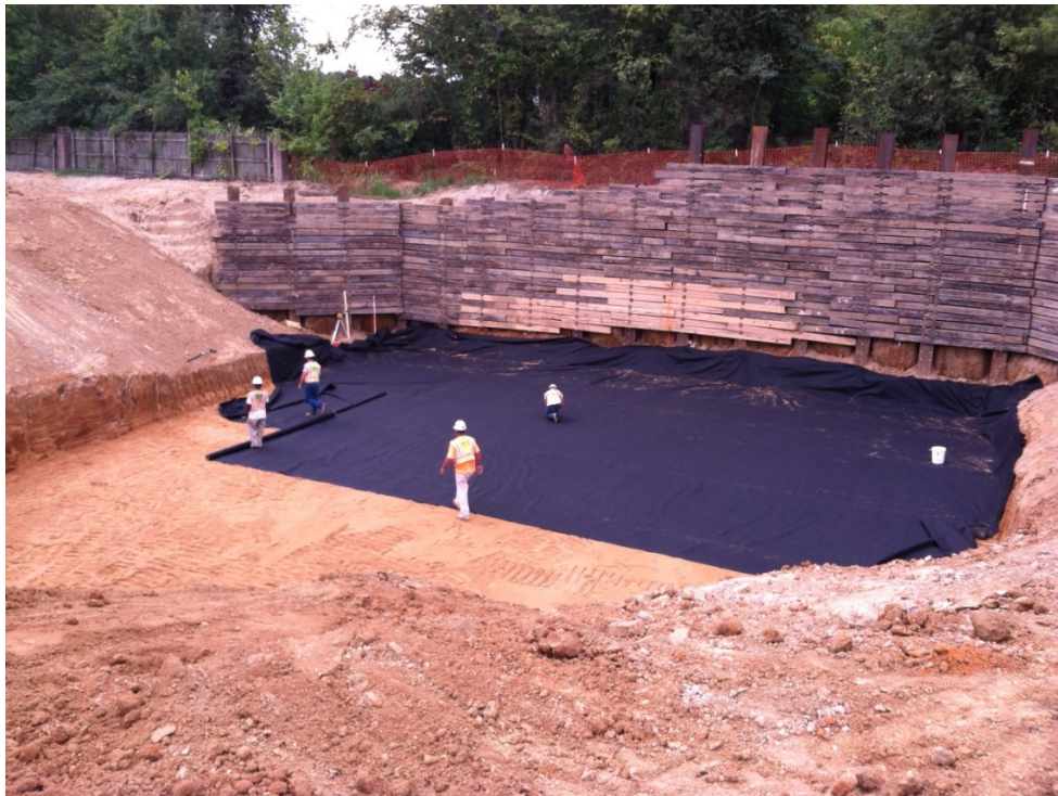
Western pond area (post-excavation) being prepared for soil flushing gallery
