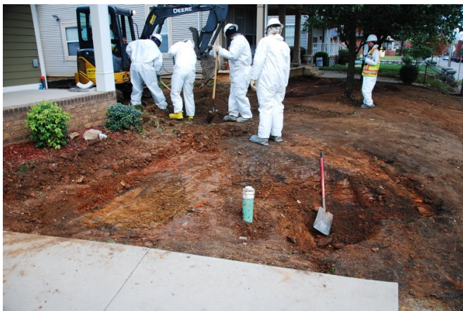
Crew conducting removal of impacted surface soil
