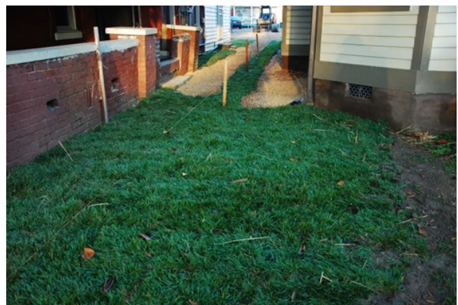
Condition of yard after remediation work completed
