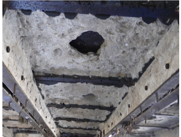
Underside of Mercury Cell Plate Bridge
