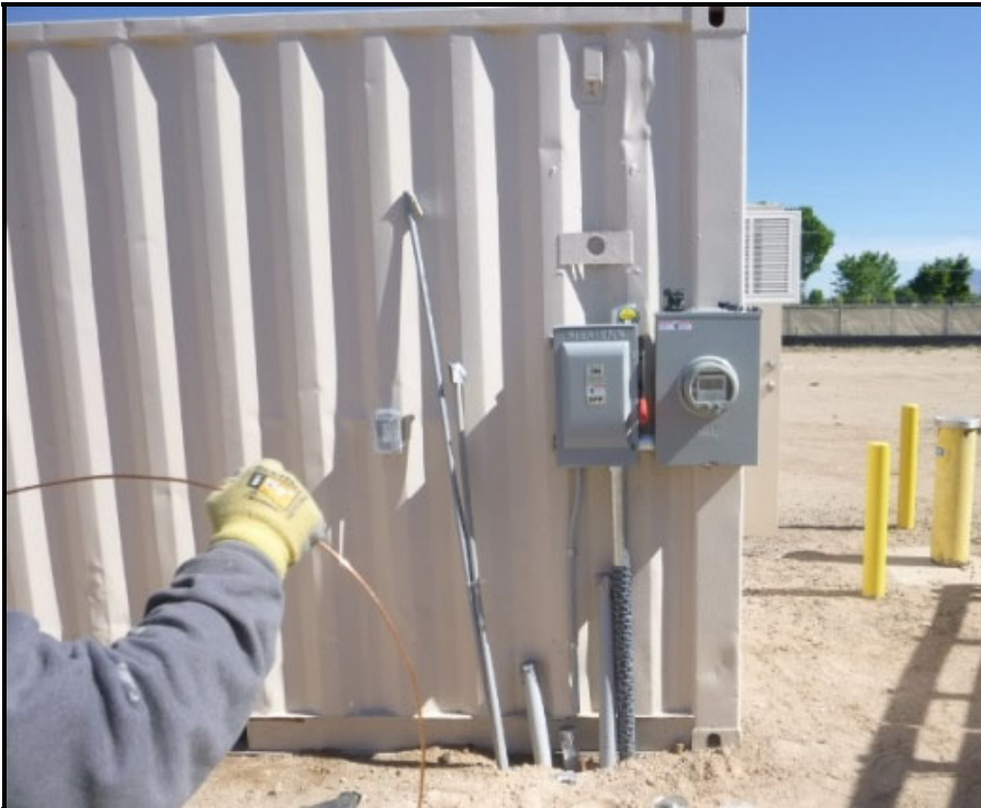
Description: Working on the main electrical disconnect and meter wiring.
