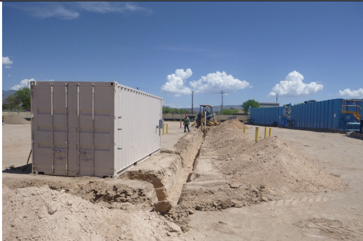
Description: Trenching to place conveyance piping.
