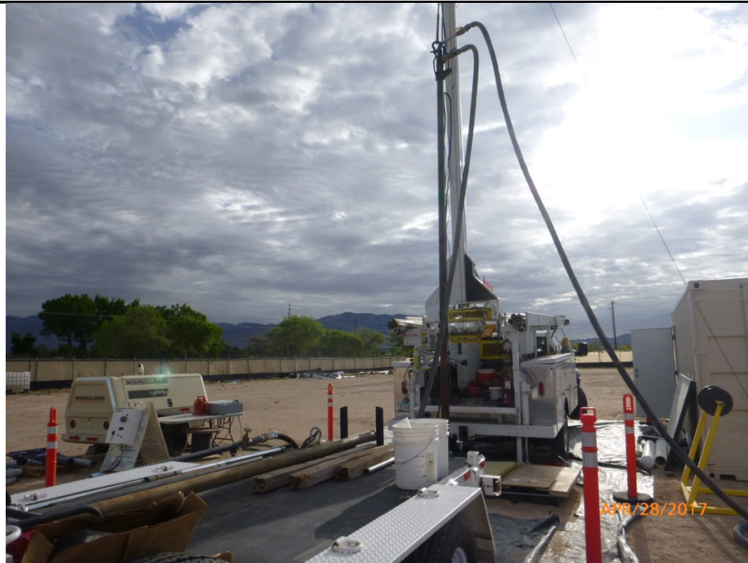
Description: Well development setup at KAFB-106IN1, with jetting tool.
