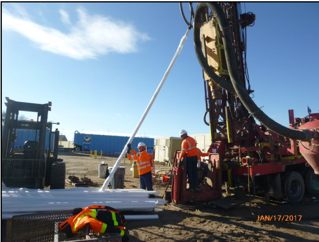
Description: Cascade installing PVC casing during well installation activities.
