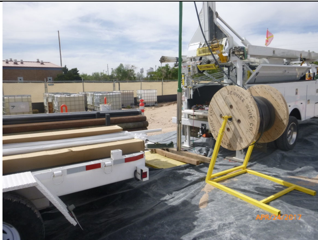
Description: Installing Grunfos pump at KAFB-106EX2.
