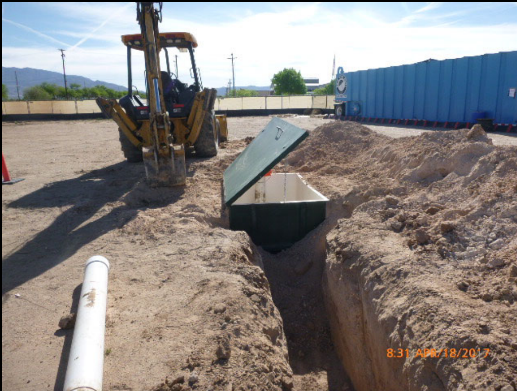
Description: Installing KAFB-106EX1 well vault and trenching for utilities/pipeline.
