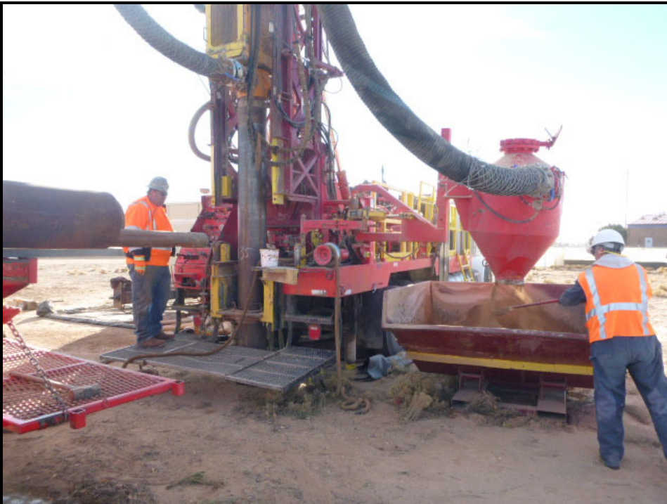
Description: Geologist collecting soil cuttings from hopper during drilling operations for lithologic classification.
