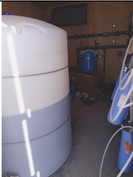
Description: Treatment amendments homogenized in tank and ready for injection.
