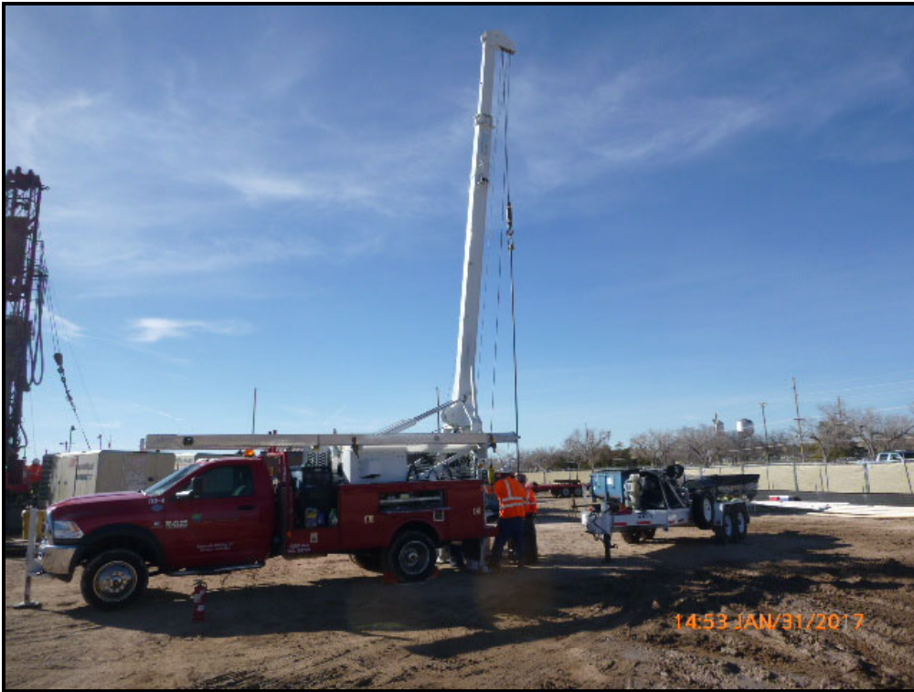
Description: Cascade well development rig setup.
