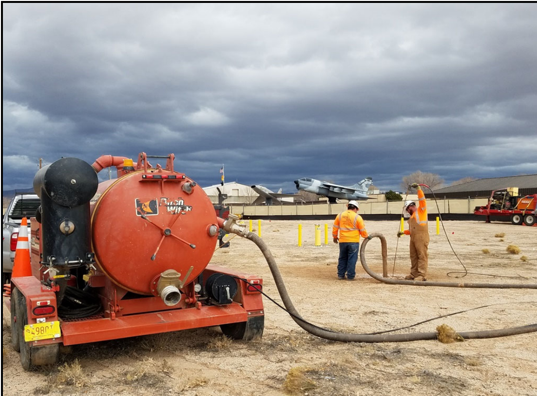
Description: High Mesa potholing for utilities at KAFB-106IN1.
