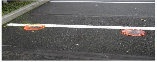
Photo 11: Groundwater Monitoring Wells W85-5A and W85-5B identified for decommissioning
